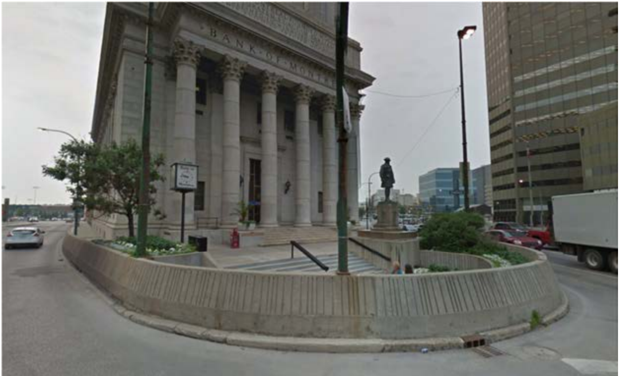
Figure 22 – Depressed Patio Area on SE corner
