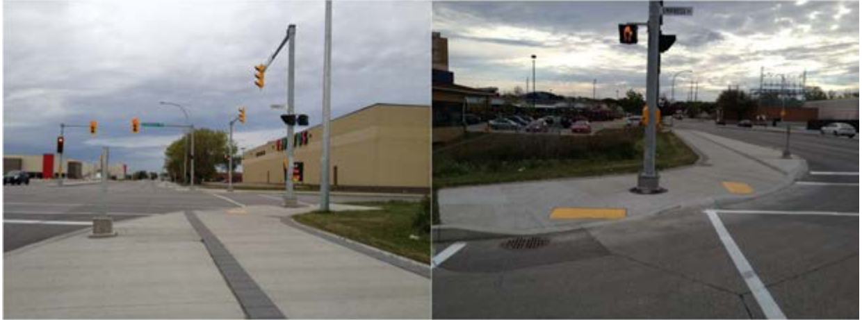
Figure 30 – Recent Roadworks – St. Matthews Avenue and Empress Street
