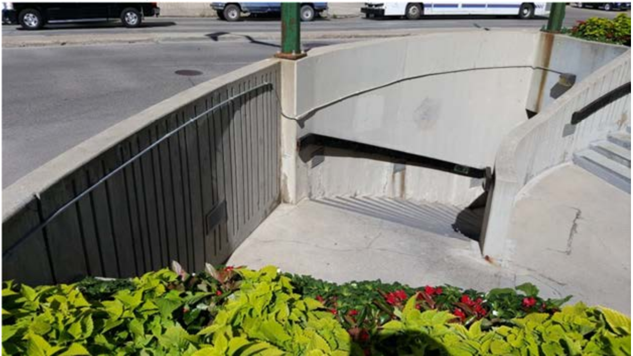
Figure 23 – Depressed Patio Area - Existing Staircase on SE corner
