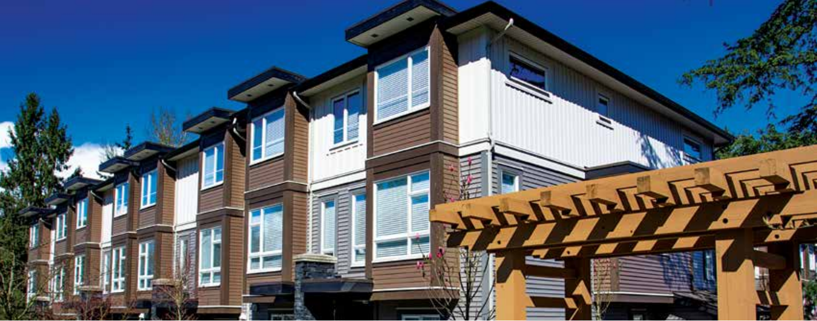
Townhouse design that utilizes projections, a mix of materials and varied roof lines to create visual interest.
