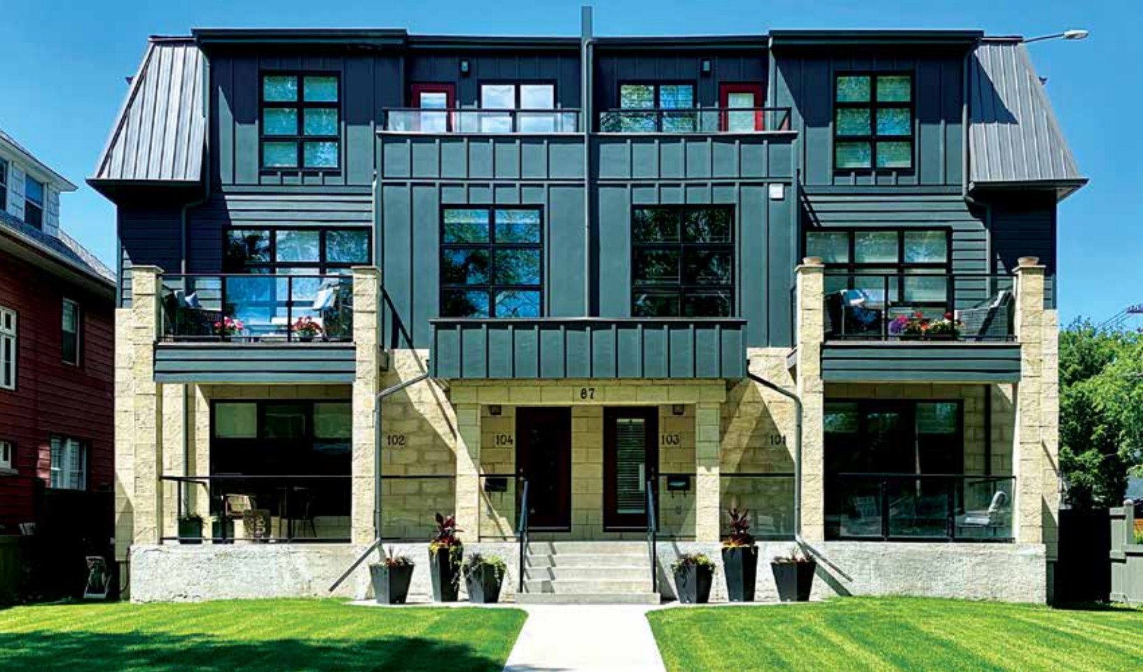
An example of a high quality design that meets the requirements for façade and architectural features.
