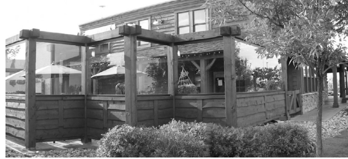
Glazing can provide some sound attenuation for patios near residential areas.
