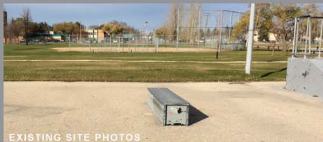
EXISTING SITE PHOTOS
