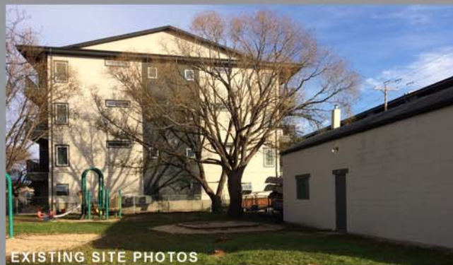
EXISTING SITE PHOTOS
