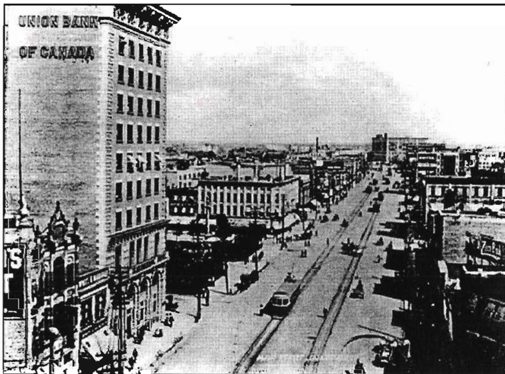
PLATE 12: Main north of William, c.1910. The effects of post-1900 development are evident when a comparison of the skyline in this scene is made with Plate 4. (PAM, Photograph Collection, Winnipeg-Streets-Main, c.1910, #4 )
