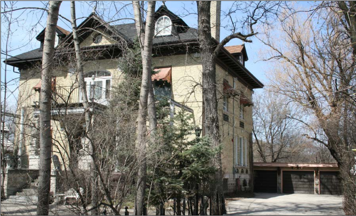
Front (south) and east façades, 2009
