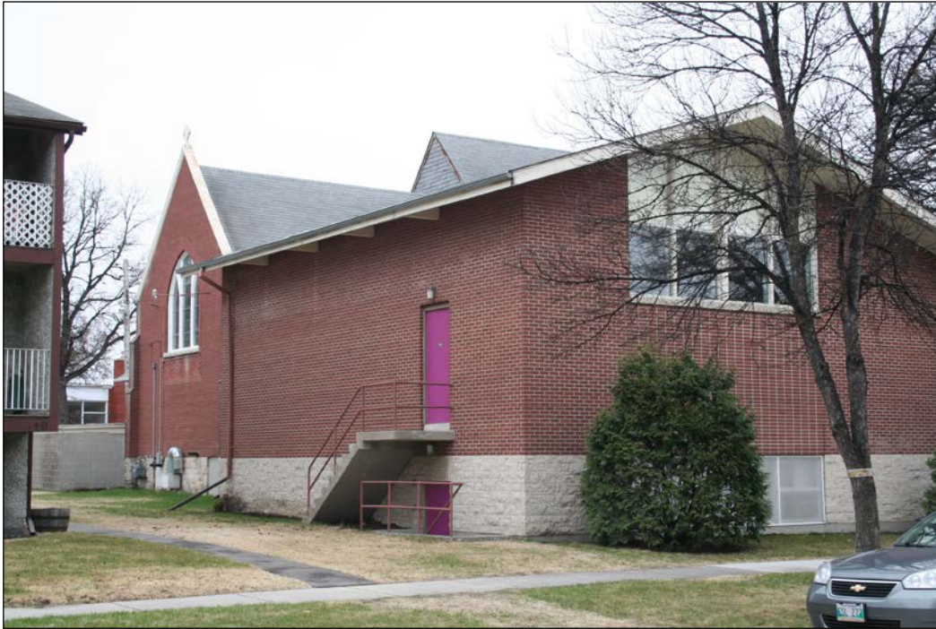
Rear (east) and north façades, 2009
