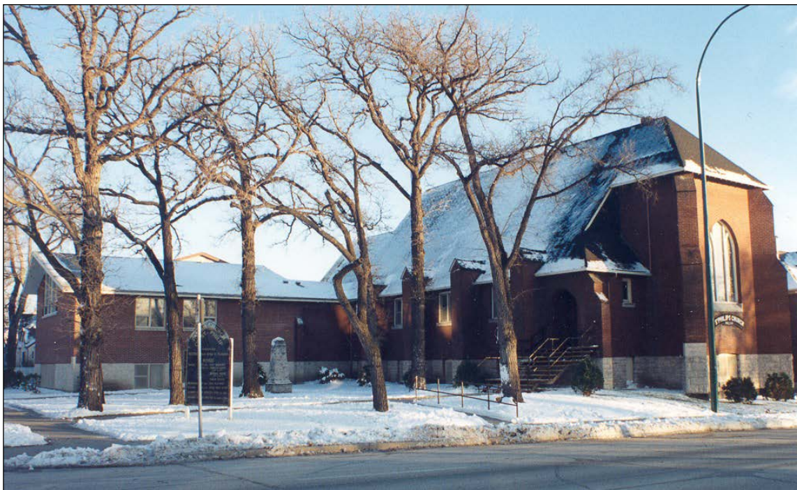
Front (west) and north façades, 1994
