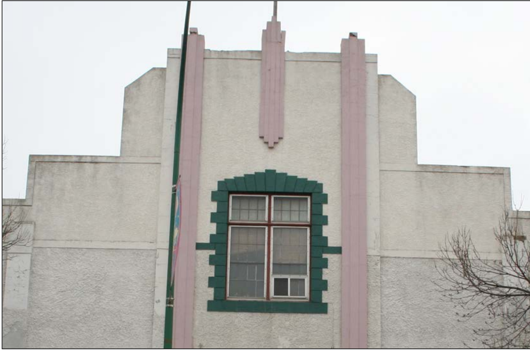
Front (south) façade detail, 2009
