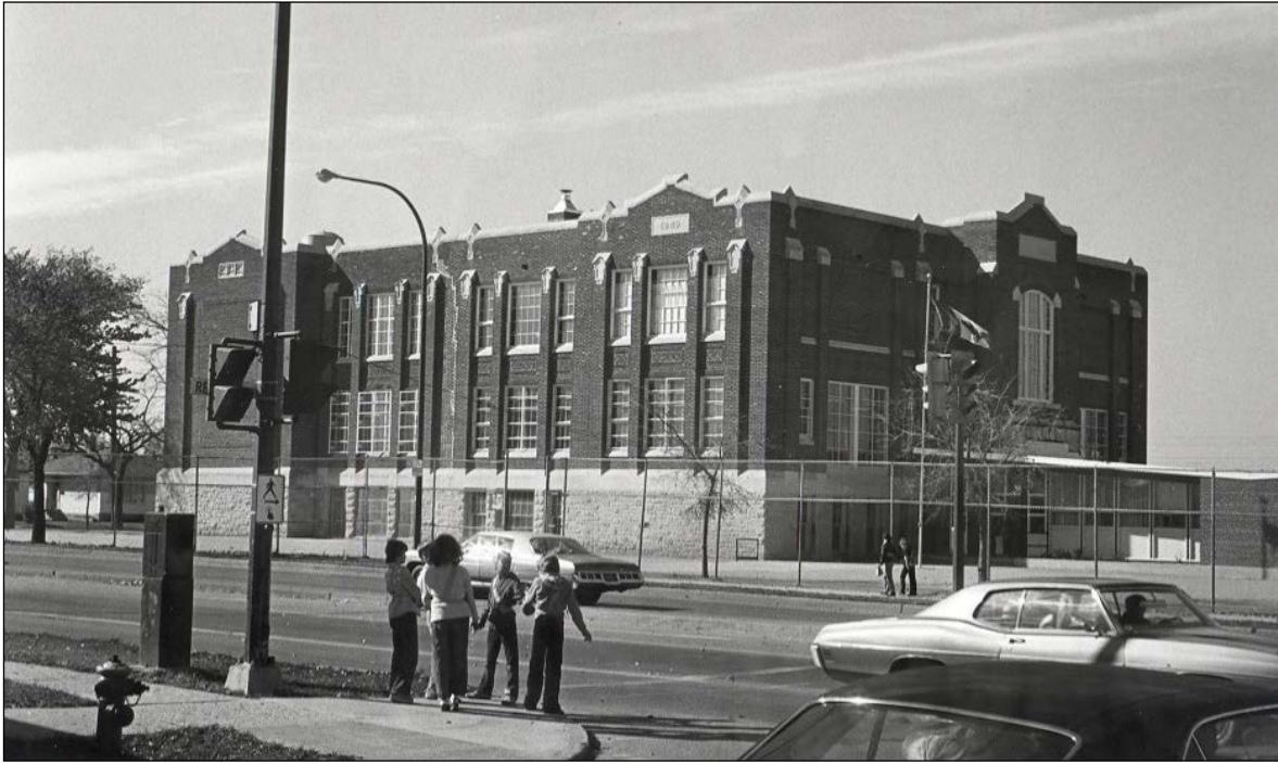
East and north façades, 1978
