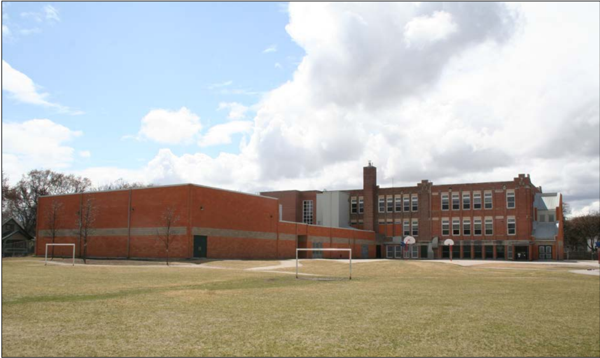
Rear (east) façade, 2009
