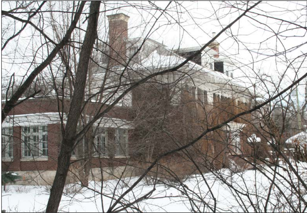
Rear (south) and west façades, 2009
