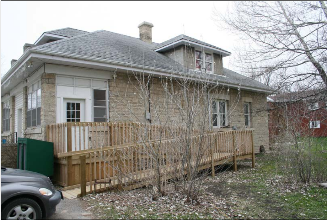
Front (east) and north façades, 2009
