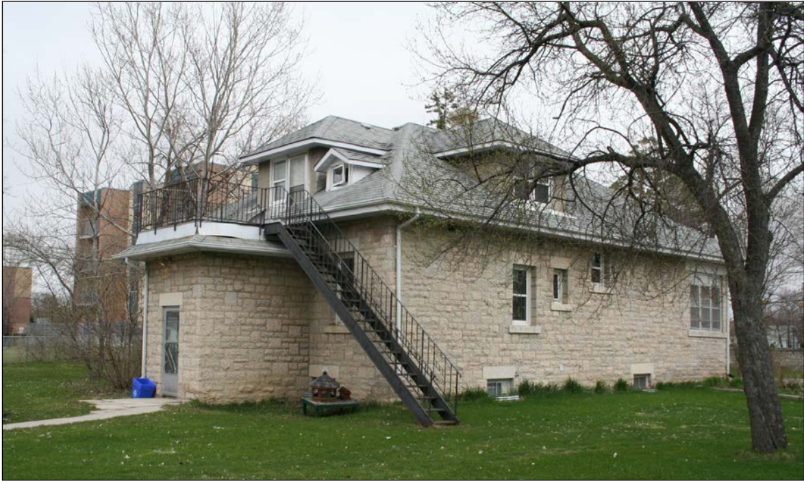
Front (east) and north façades, 1978
