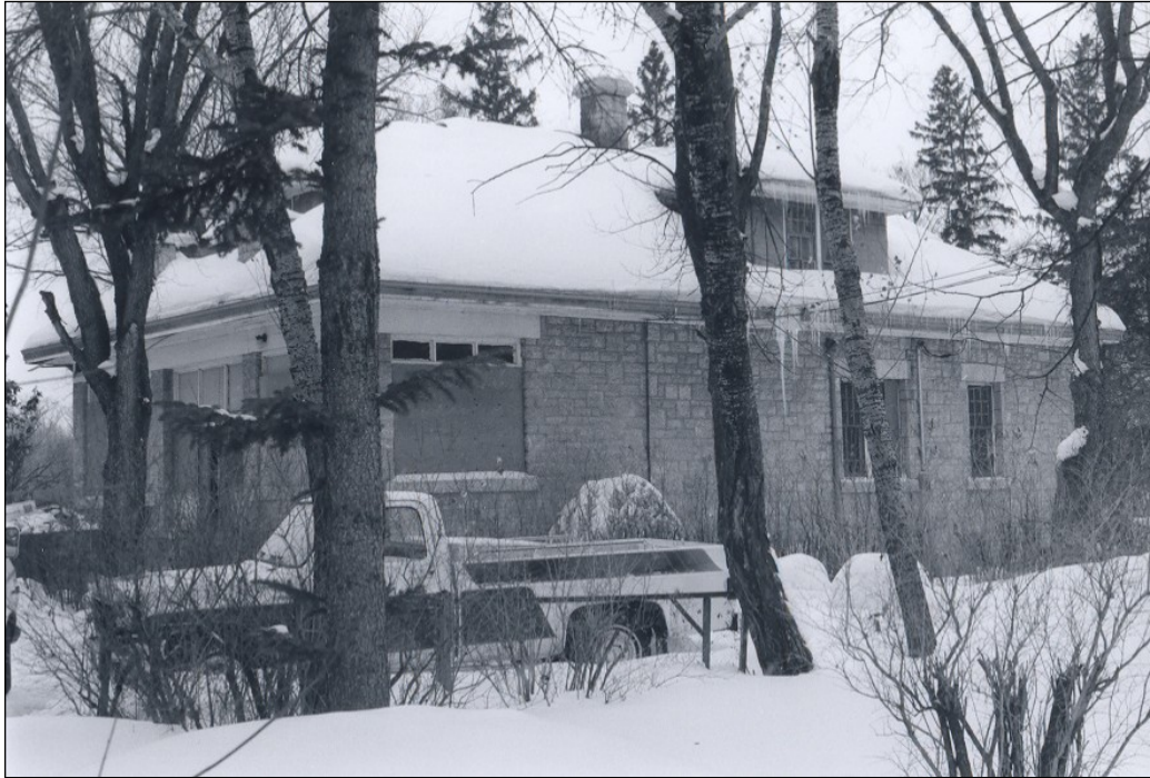
Front (east) and north façades, 1978
