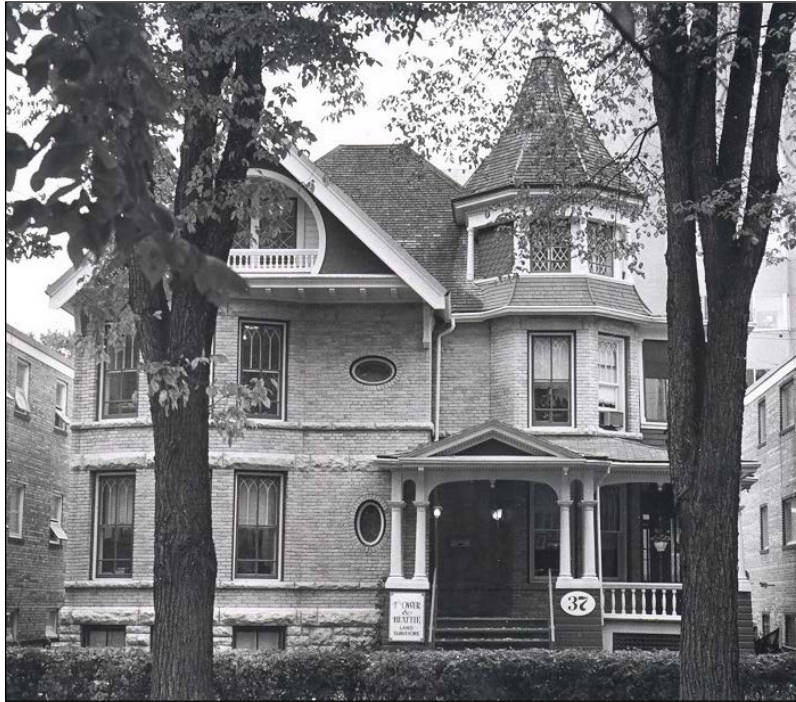
Front (west) façade, 1978.
