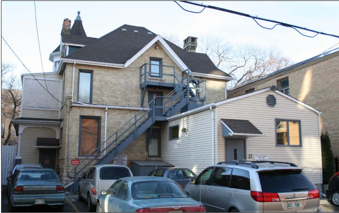
Rear (east) and south façades, 2006.
