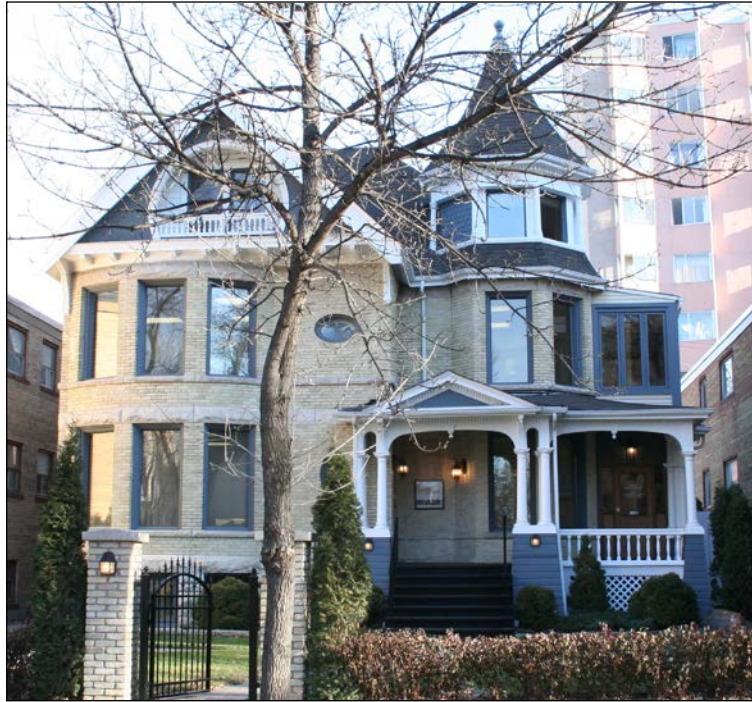
Front (west) façade, 2006.
