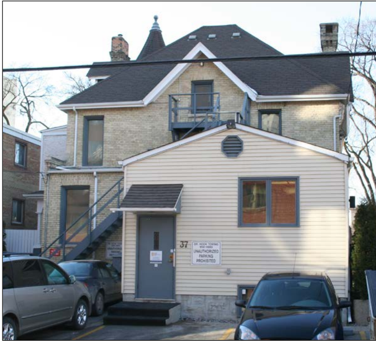
Rear (east) façade, 2006.
