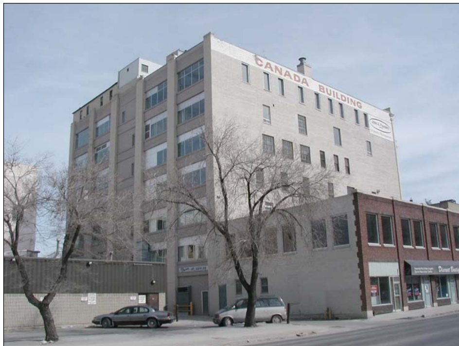
Plate 6 – Canada Building, rear (west) and south sides. ( M. Peterson, 2003. )
