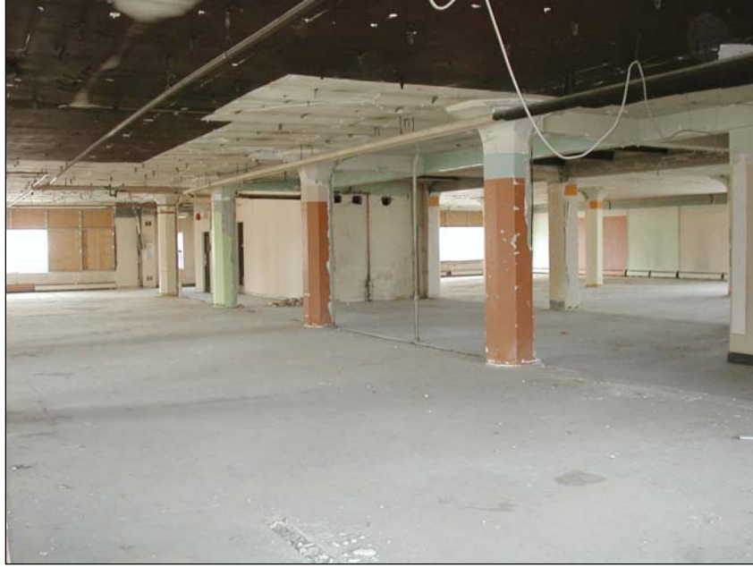
Plate 9 – Canada Building, fourth floor. ( M. Peterson, 2003. )
