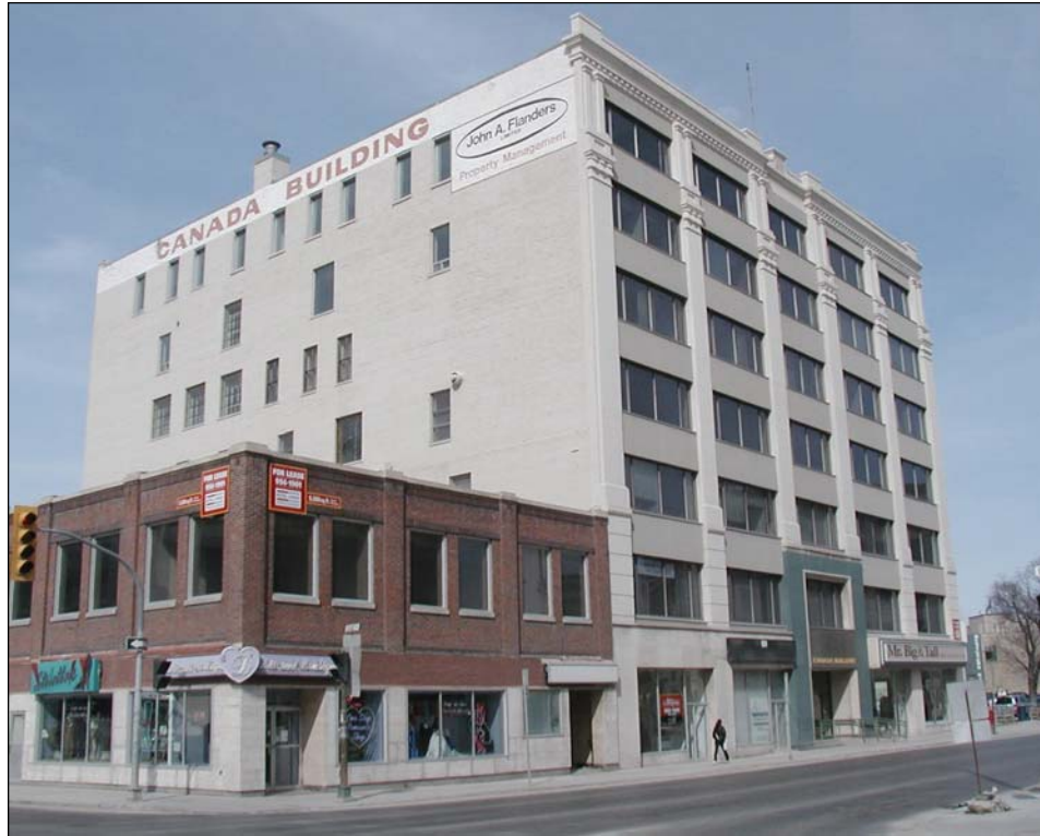
Plate 5 – Canada Building, front (east) and south sides. ( M. Peterson, 2003. )
