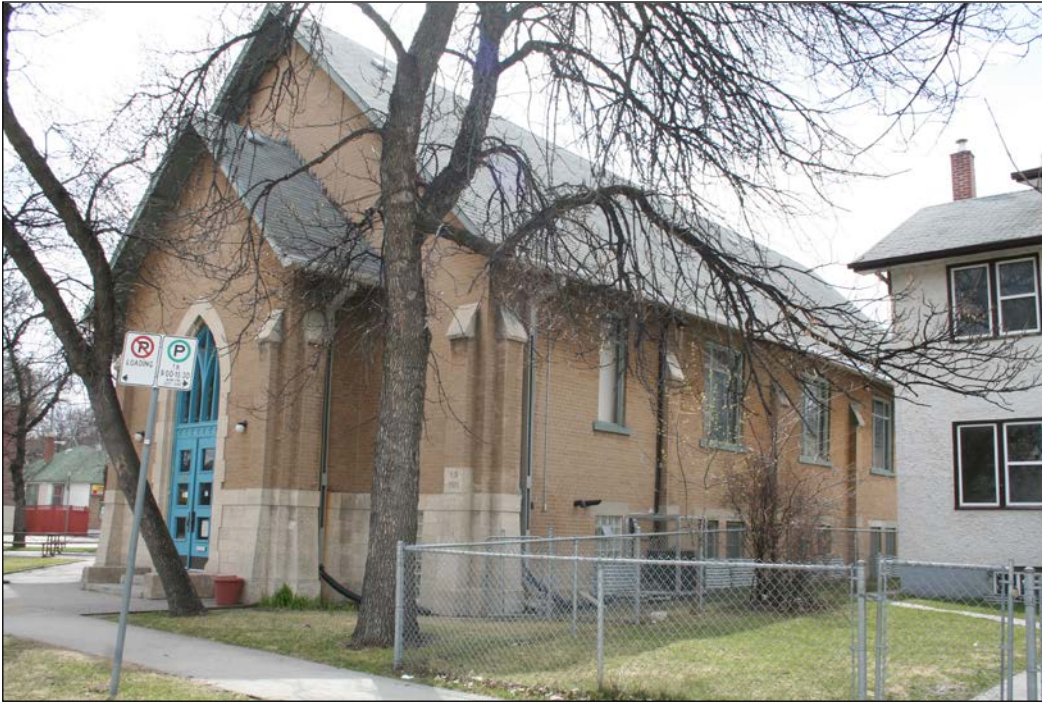
Front (east) and north façades, 2009
