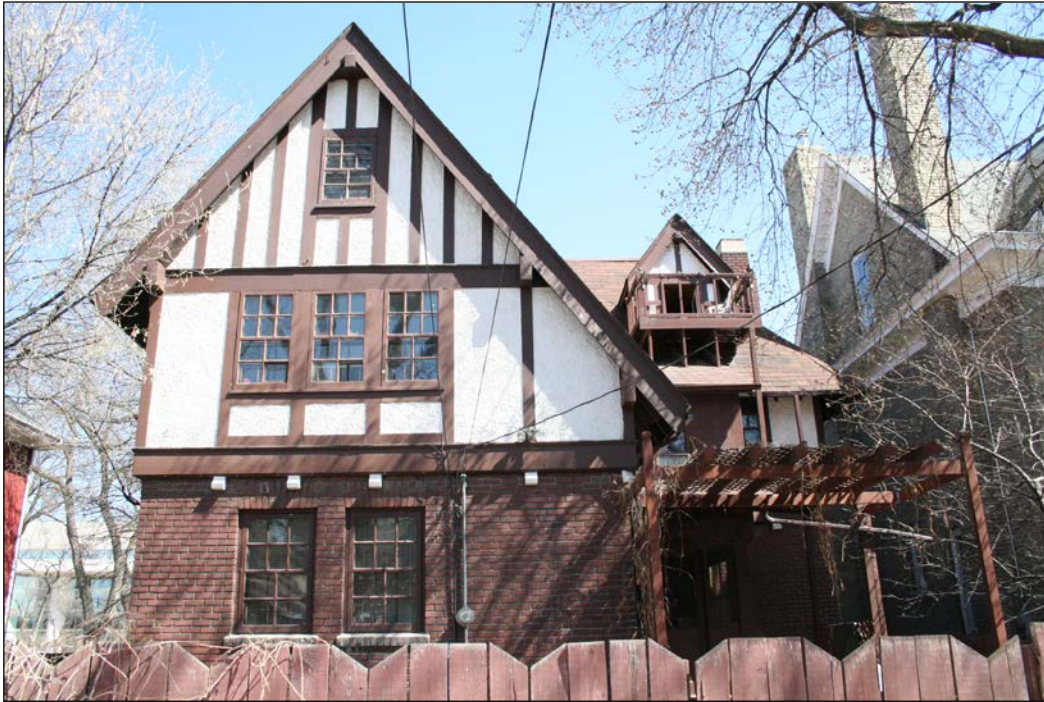
Rear (west) façade, 2007
