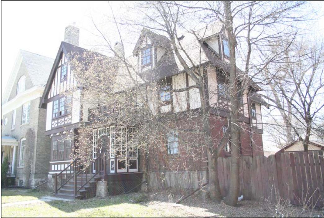
Front (east) and north façades, 2007
