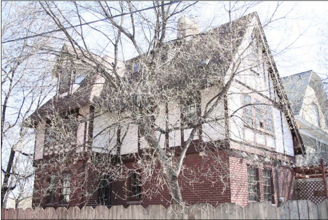
Rear (west) and north façades, 2007
