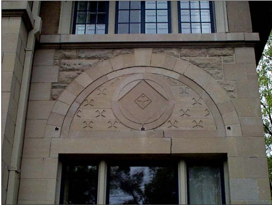
Front (south) façade detail, 2000
