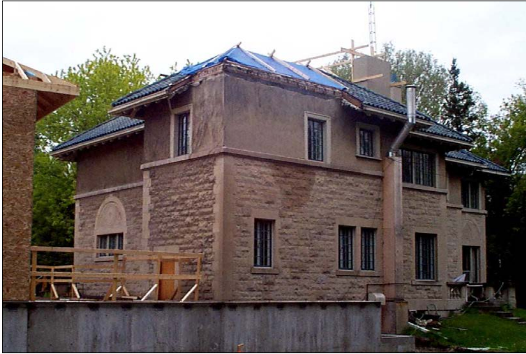
Rear (north) and east façade, 2000
