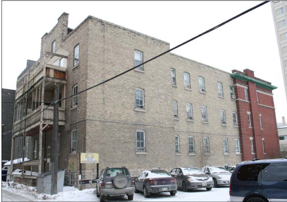
Rear (west) and south façades, 2006
