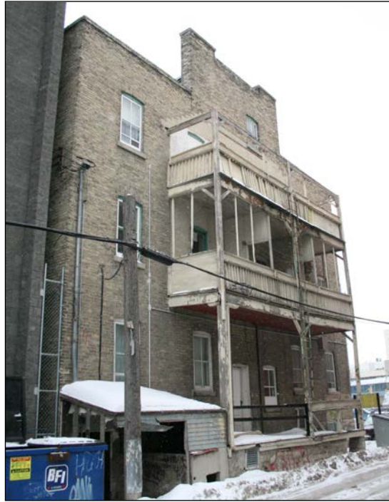
Rear (west) façade, 2006
