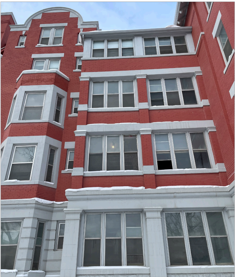
Roslyn Apartments, 40 Osborne St., typical windows, 2024
