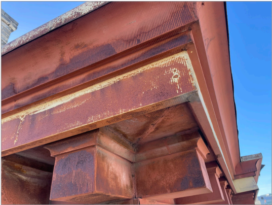
Peck Building, 33 Princess St., metal cornice, northeast corner, Hi-Rise Limited, 2026
