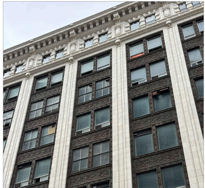
Boyd Building, 388 Portage Ave., east façade detail, 2025
