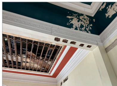
Carnegie Library, 380 William Ave., renovation work continues, 2026
