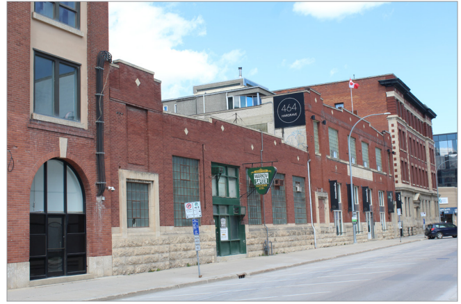
West side of Hargrave Street, south of McDermot Avenue, including 462 & 464 Hargrave St., 2025
