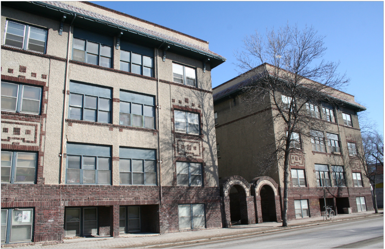
Gaspé Apartment and Annex, 597-601 Broadway, 2009
