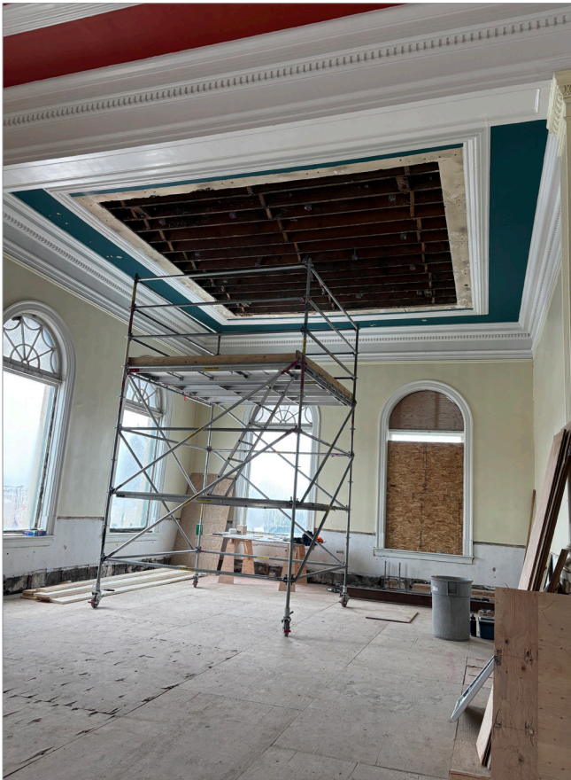
Carnegie Library, 380 William Ave., renovation work continues, 2026
