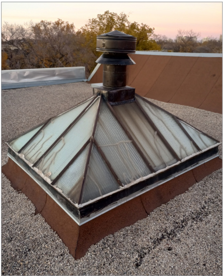
Thelma Apartments, 272 Home St., skylight, 2025
