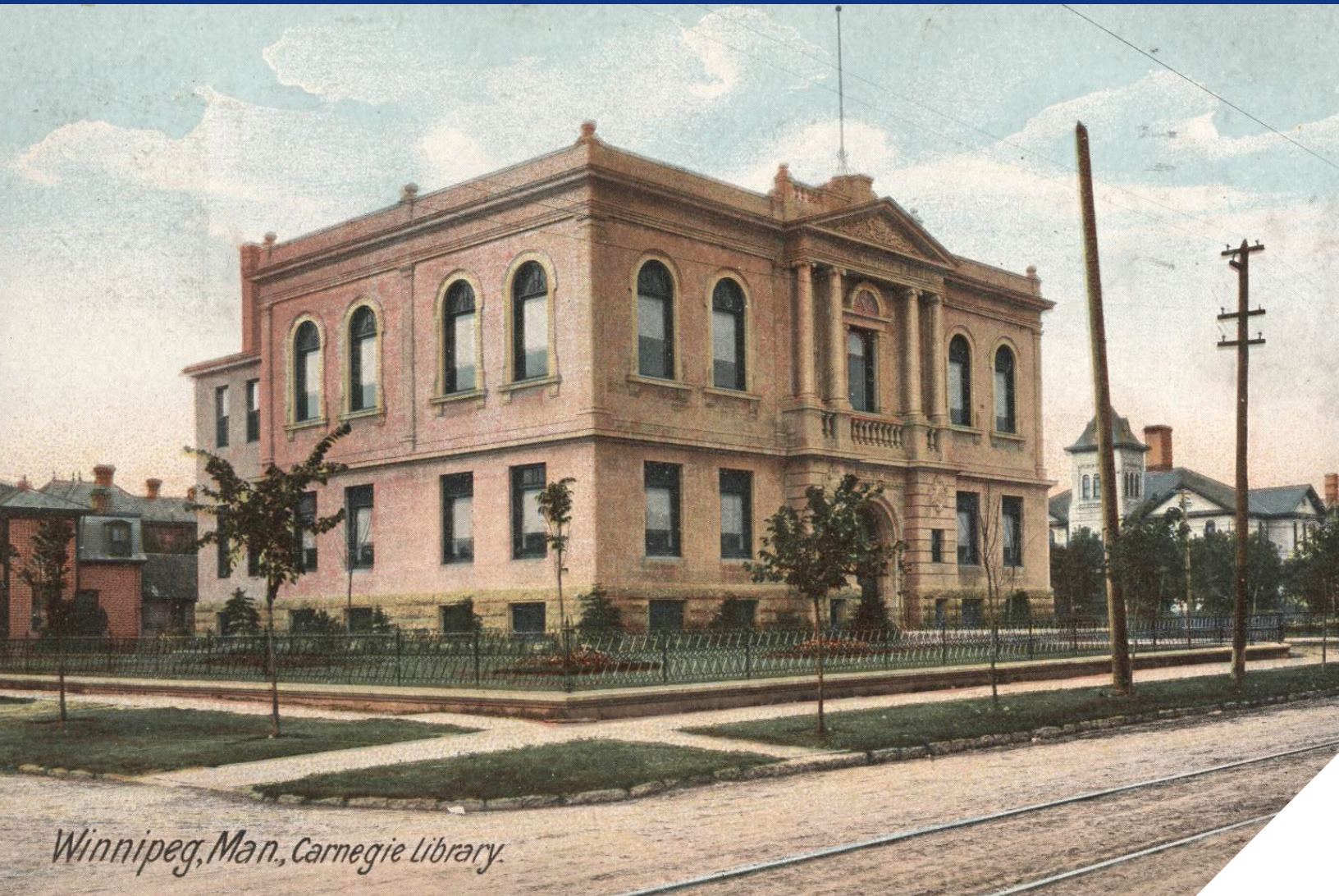
Undated colour postcard of the Carnegie Library, now the City of Winnipeg Archives Building, 380 William Ave., which is undergoing extensive renovations and upgrades
