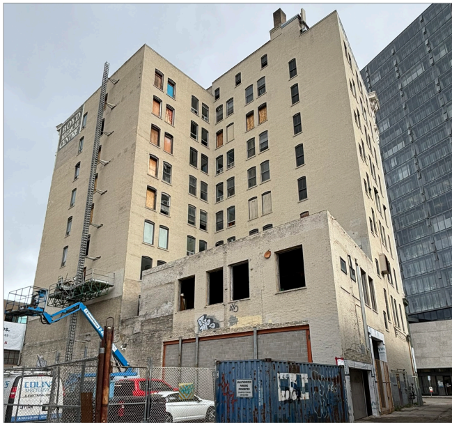
Boyd Building, 388 Portage Ave., rear window replacement, 2025
