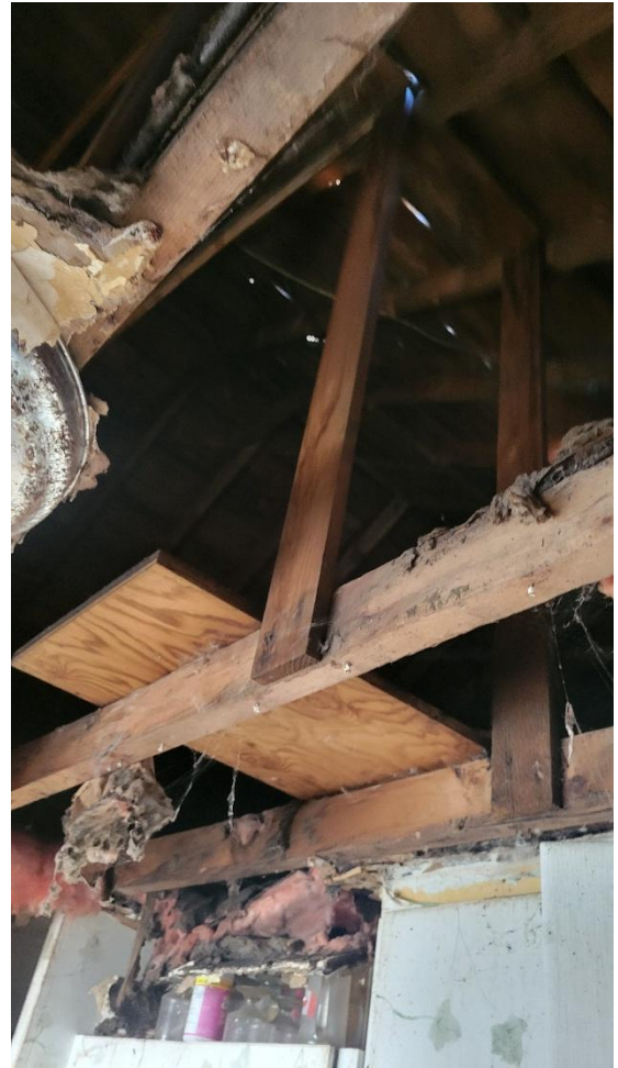
Portion of Ceiling
