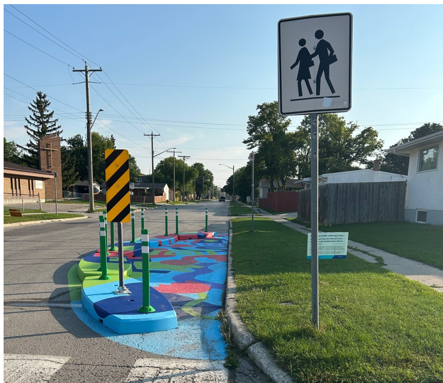
Calming curb on Watt Street Photo Credit: City of Winnipeg
