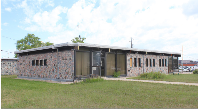
Windsor Park Library, 955 Cottonwood Rd., front and west façades, 2021
