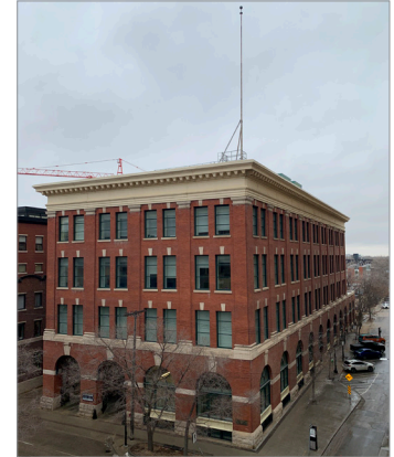
Customs Examining Warehouse, 145 McDermot Ave., west and south façades, 2024
