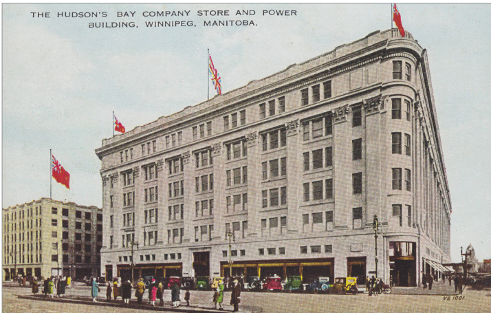
Hudson's Bay Company Building, 450 Portage Ave., date unknown. Winnipeg Public Library, Rob McInnes Post Card Collection number 4835
