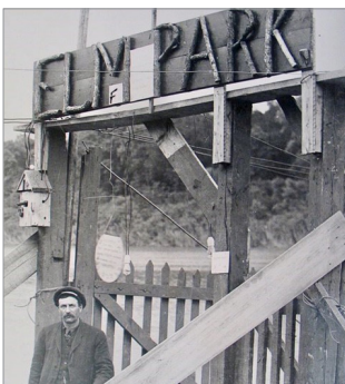
Elm Park pontoon bridge entrance, date unknown
