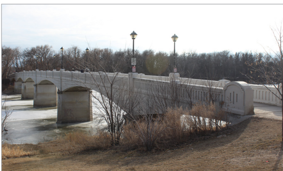
Assiniboine Park Footbridge, east side, 2021
