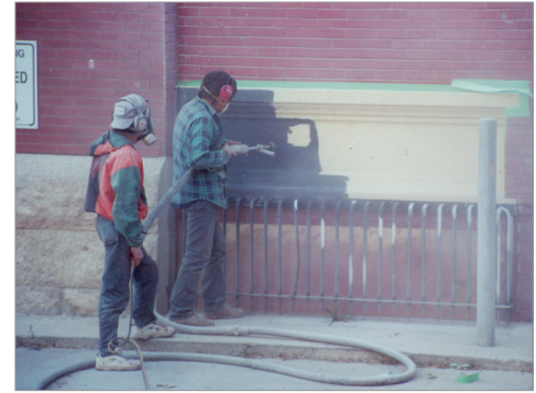
Customs Examining Warehouse, 145 McDermot Ave., sand blasting the metal to remove paint, 2000
