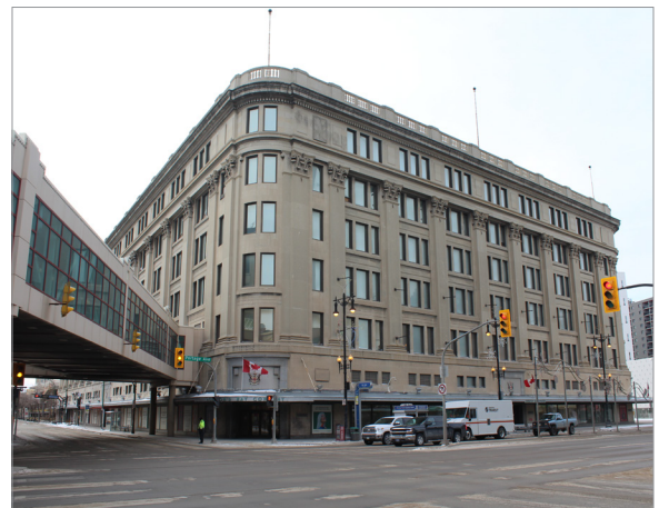
450 Portage Ave., Hudson's Bay Company Building
