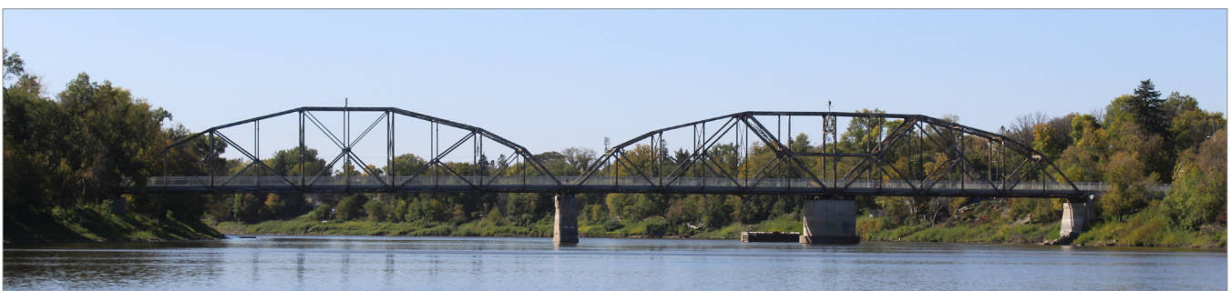
Elm Park Bridge, west side, 2022
