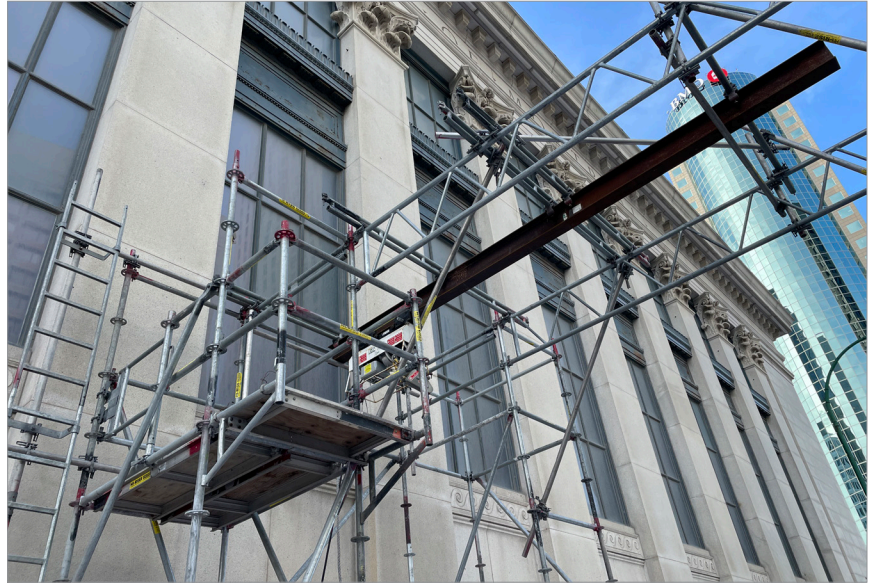
335 Main St., work continuing on the front façade, 2024
