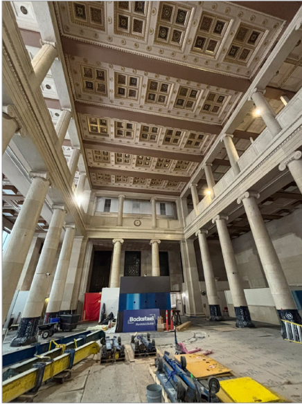
335 Main St., former banking hall, 2025
