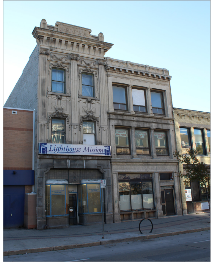
667 & 669 Main St., front façades, 2018
