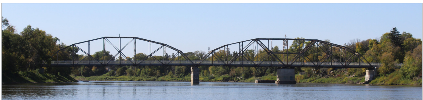
Elm Park Bridge, west side, 2022
