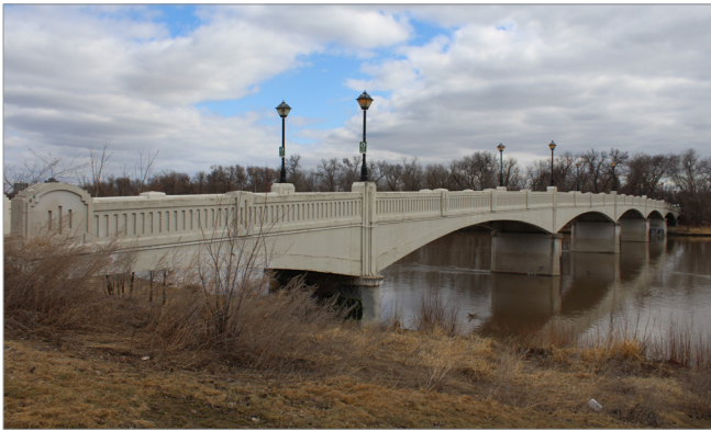
Assiniboine Park Footbridge, west side, 2023
