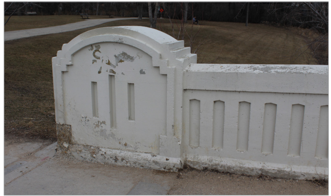
Assiniboine Park Footbridge, detail, 2023
