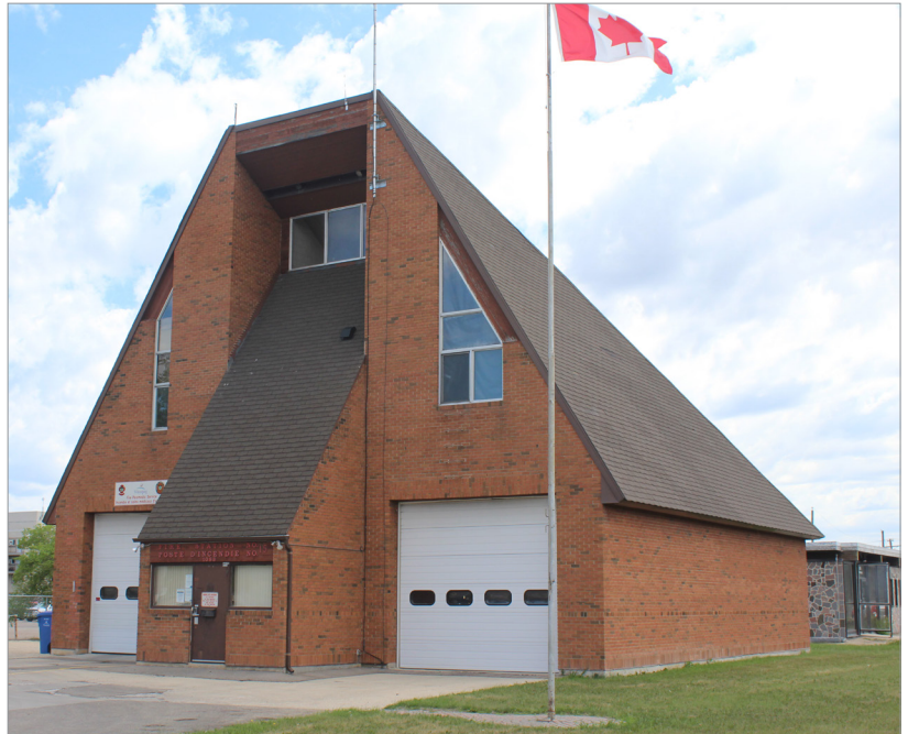
Fire Station No. 4, 1083 Autumnwood Dr., front and south façades, 2021
