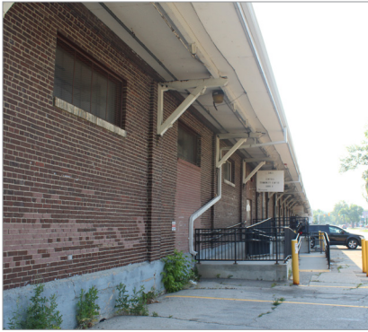
Midland Railway Building, 200 Isabel St., south façade, 2021
