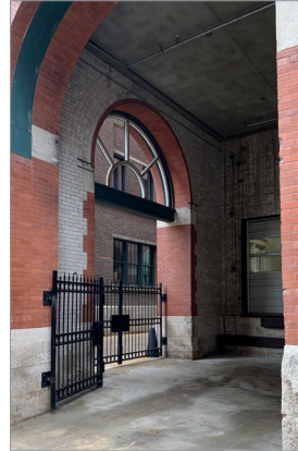
Customs Examining Warehouse, 145 McDermot Ave., northwest corner with metal grates, 2024
