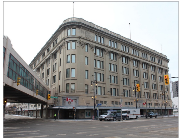
450 Portage Ave., Hudson's Bay Company Building
