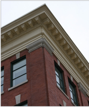
Customs Examining Warehouse, 145 McDermot Ave., roof detail, 2005
