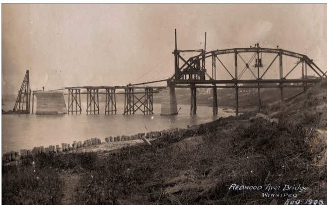
Redwood Bridge, construction work on the superstructure, August 1908
