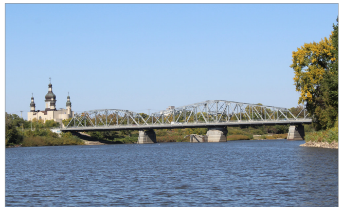
Redwood Bridge, south side, 2022
