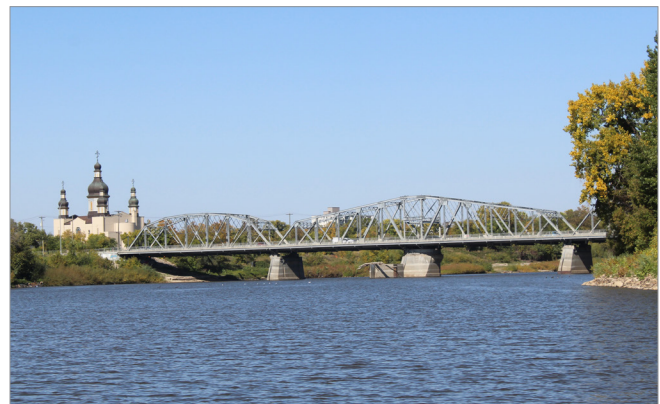
Redwood Bridge, south side, 2022
