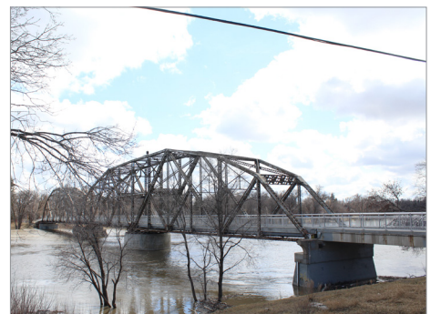
Elm Park Bridge, east side, 2023
