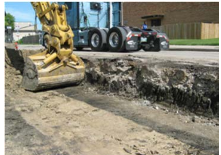
Logan Avenue Reconstruction
