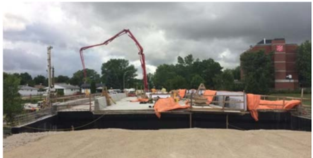
Replacement of Ness Bridge over Sturgeon Creek
