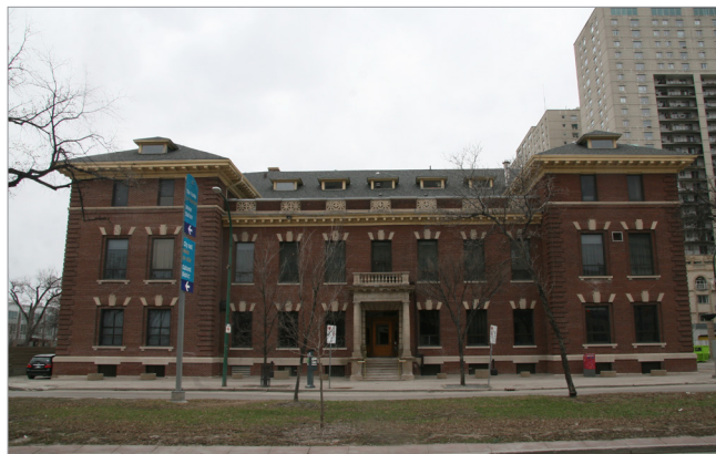
194 Broadway, Manitoba Club, façade avant (nord), 2019
