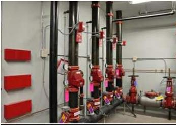
The sprinkler system is a wet system which covers the whole building. The main control valve is in the basement mechanical room.
