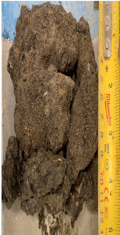
Figure 9 – Core 40 (Groverdale Ave)
