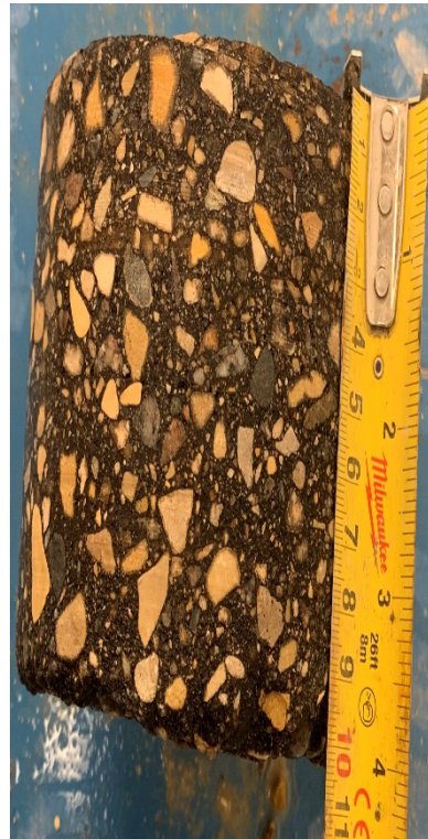
Figure 10 – Core 41 (Groverdale Ave)
