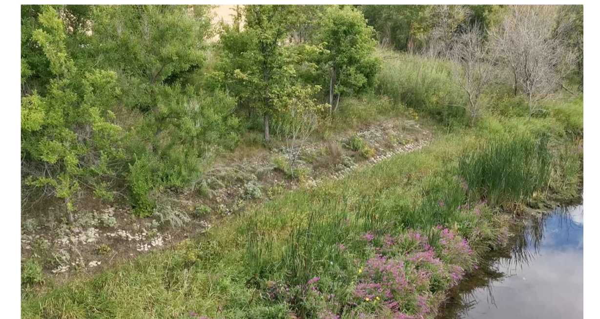
EXISTING TURFSTONE/TRI-LOCK REVETMENT SCALE N/A
