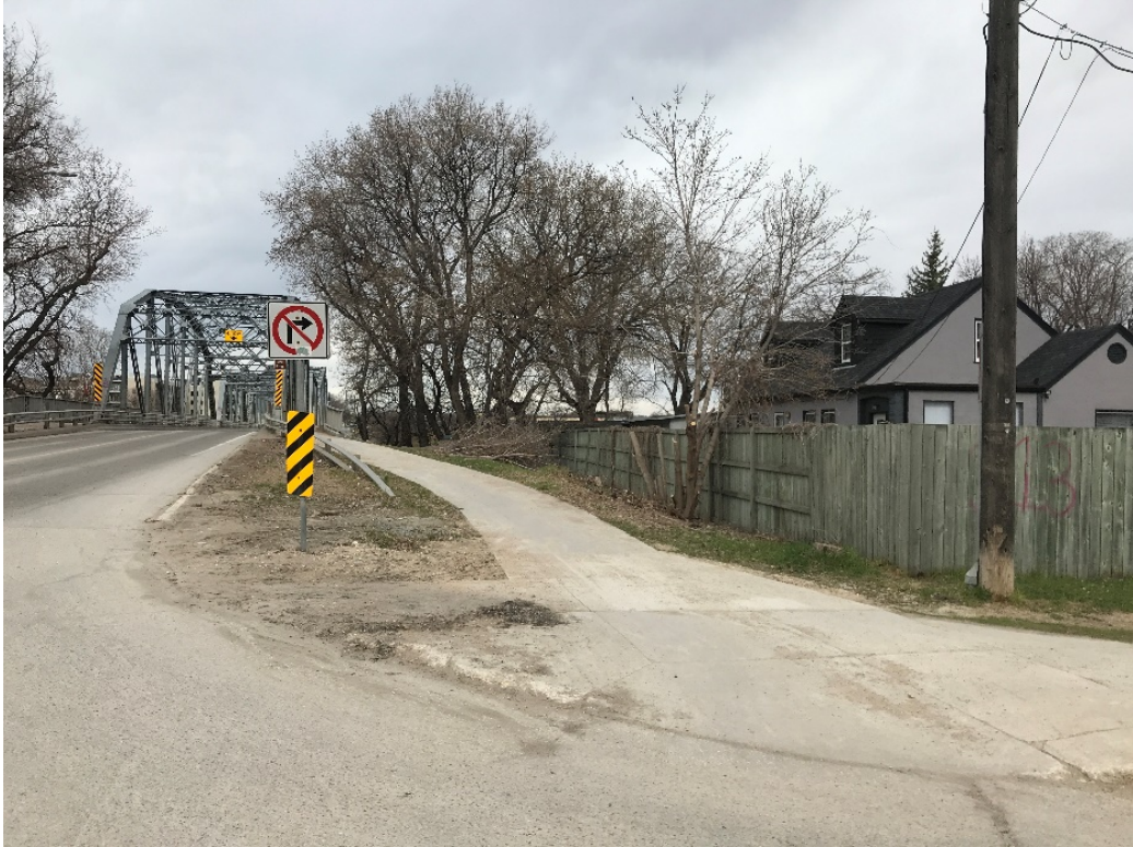
East Side - Looking west towards existing valve chamber
