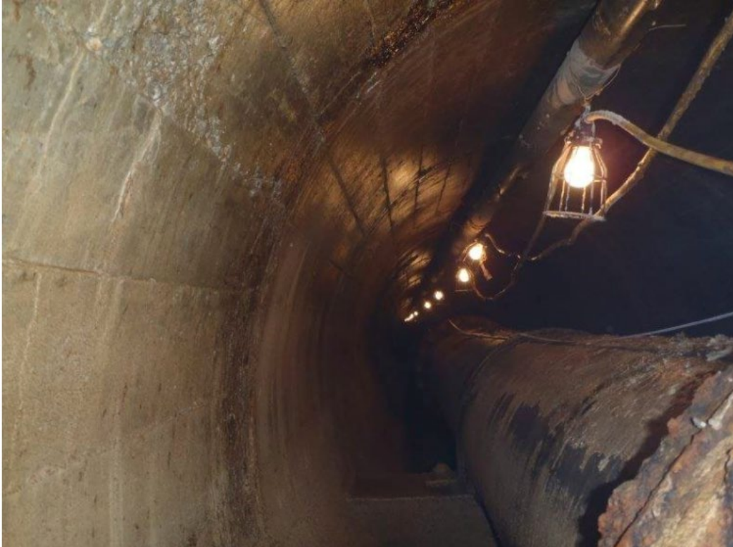
West Side – Tunnel and 600 mm feeder main
