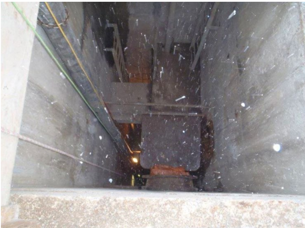
West Side - Existing tunnel shaft
