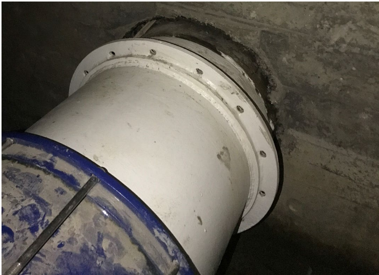
East Side – Existing valve chamber - 600 feeder main (exterior)
