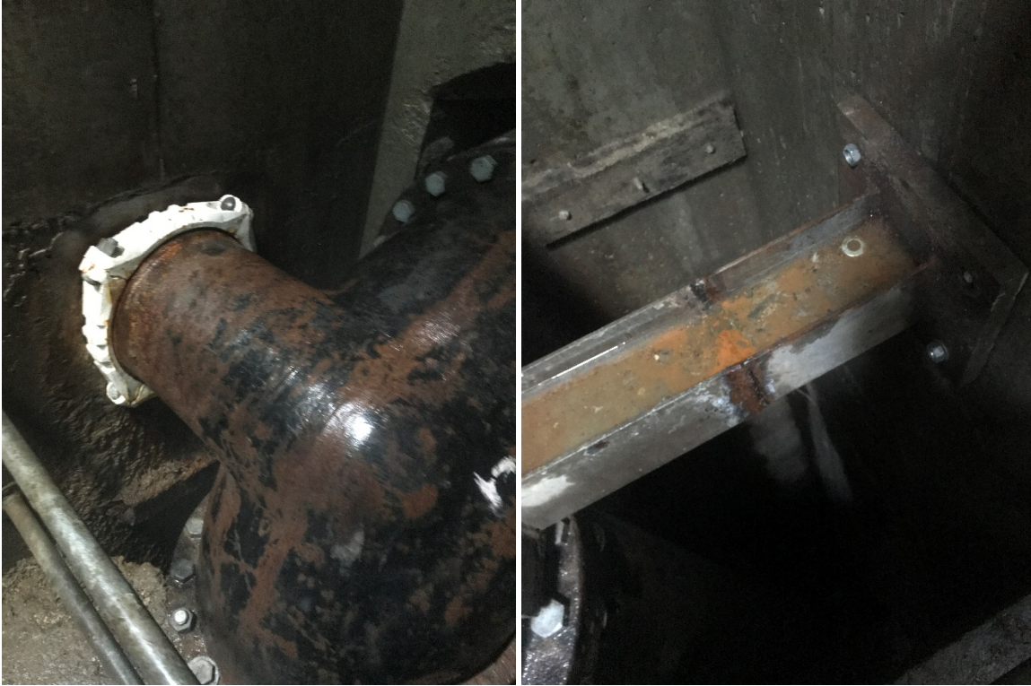
West Side – Existing tunnel shaft - Side-outlet elbow
