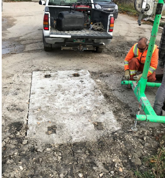
West Side – Existing tunnel shaft removable roof slab
