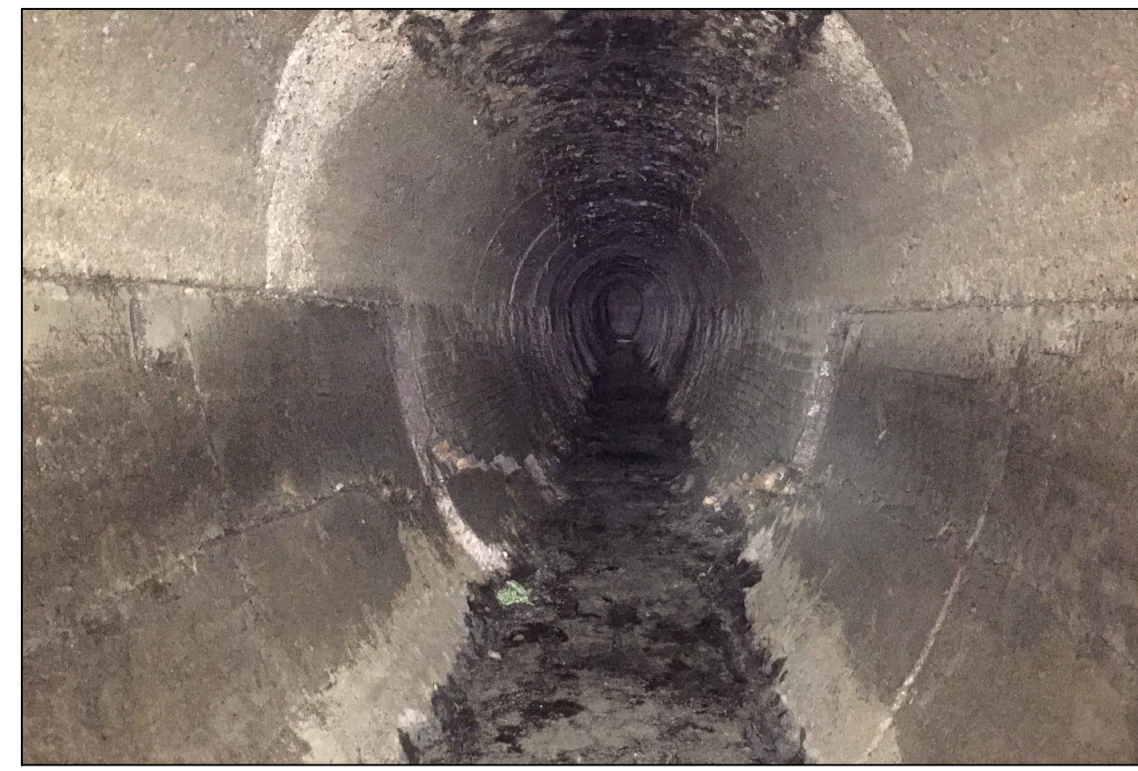
EXISTING PIPE @ APPROX. STA 1+05.0 (LOOKING UPSTREAM)
