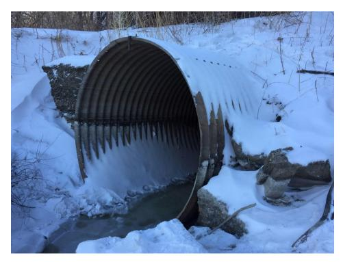
Photo 3: Close-up of outfall showing invert above the winter ice level.
