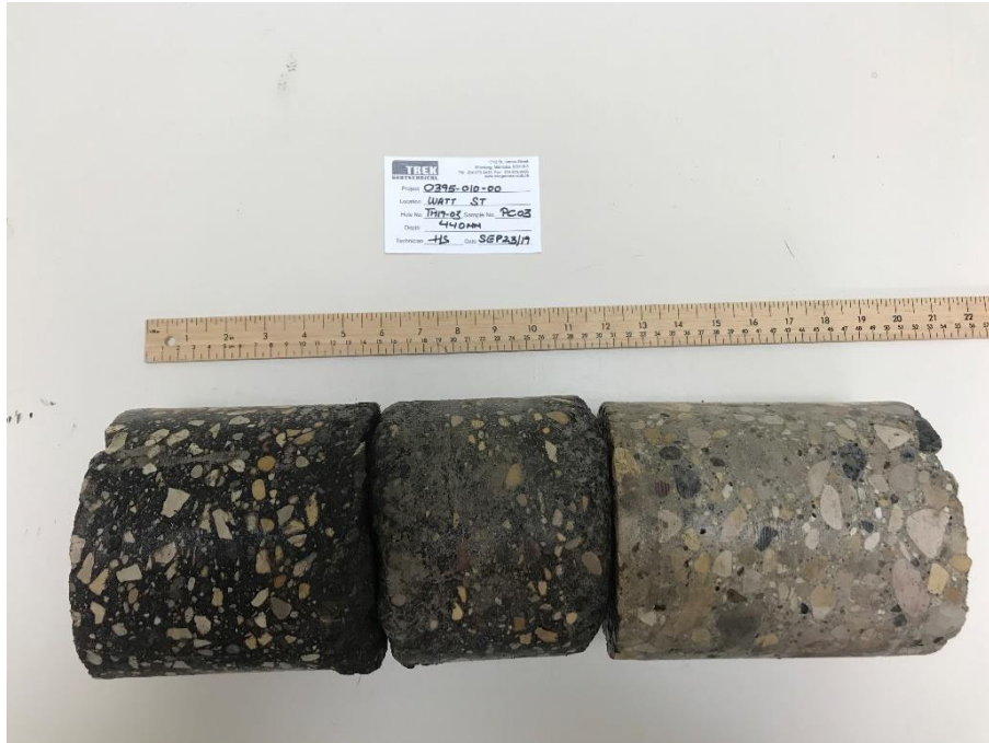
Photo 3: Pavement Core Sample at Test Hole TH19-03
