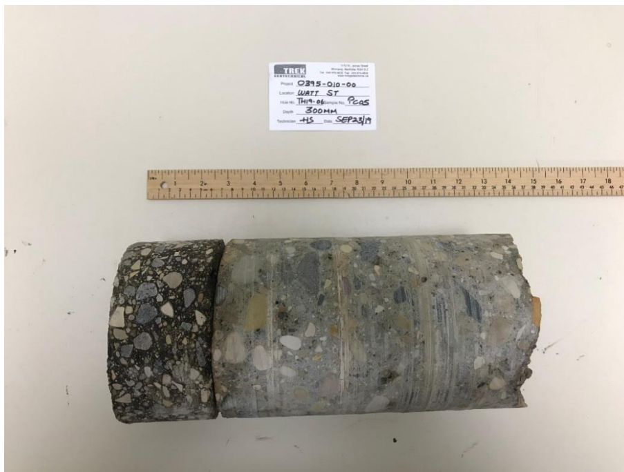
Photo 6: Pavement Core Sample at Test Hole TH19-06
