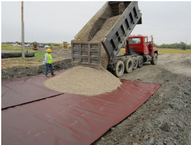
Image 3 – End dumping aggregate
