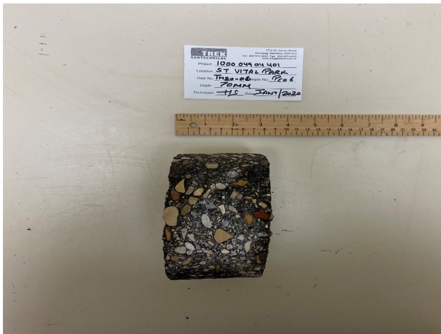
Photo 6: Pavement Core Sample at Test Hole TH20-06
