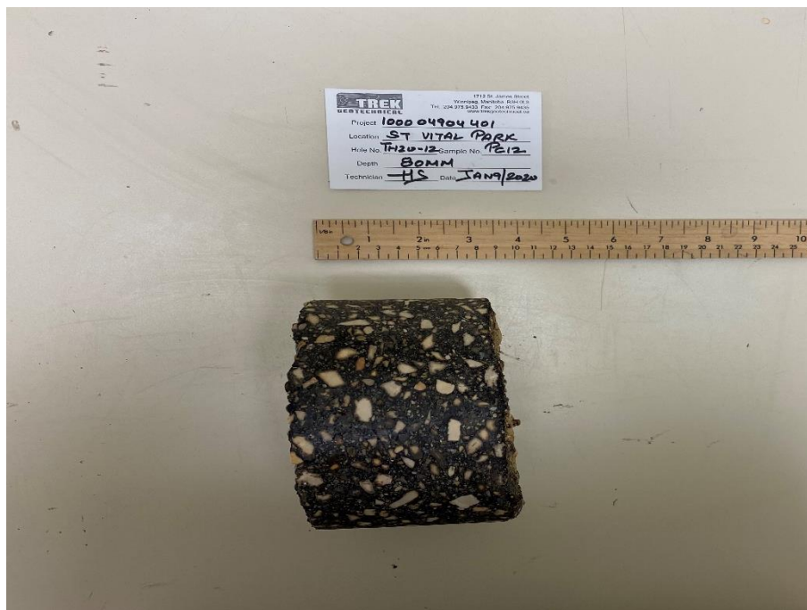
Photo 12: Pavement Core Sample at Test Hole TH20-12
