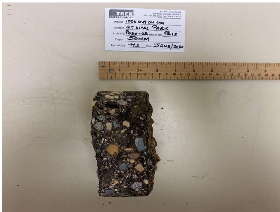
Photo 2: Pavement Core Sample at Pavement Hole PC20-02
