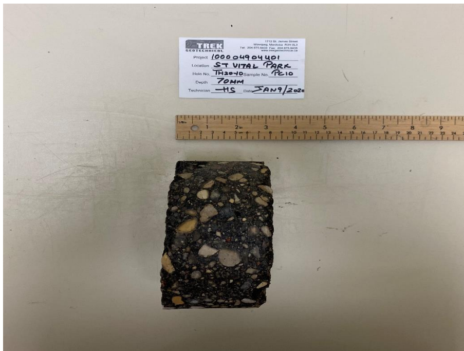
Photo 10: Pavement Core Sample at Test Hole TH20-10
