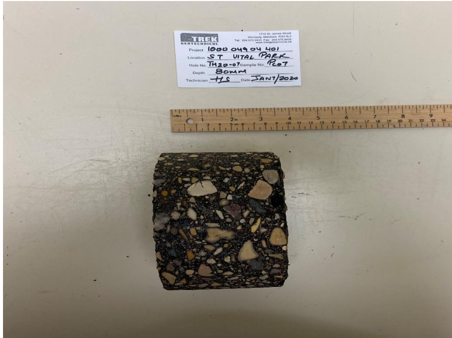
Photo 7: Pavement Core Sample at Test Hole TH20-07
