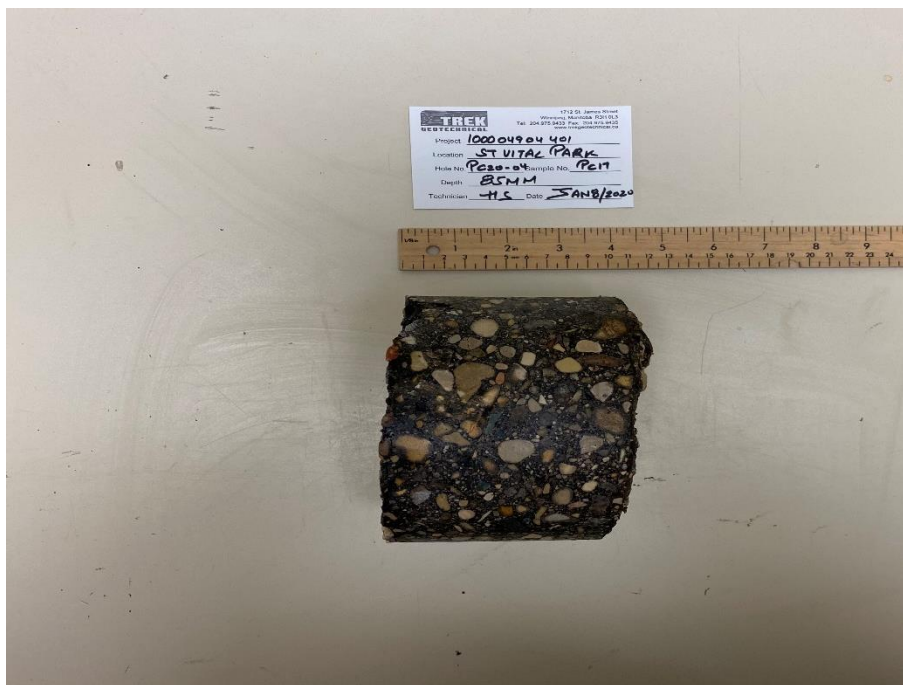
Photo 4: Pavement Core Sample at Pavement Hole PC20-04
