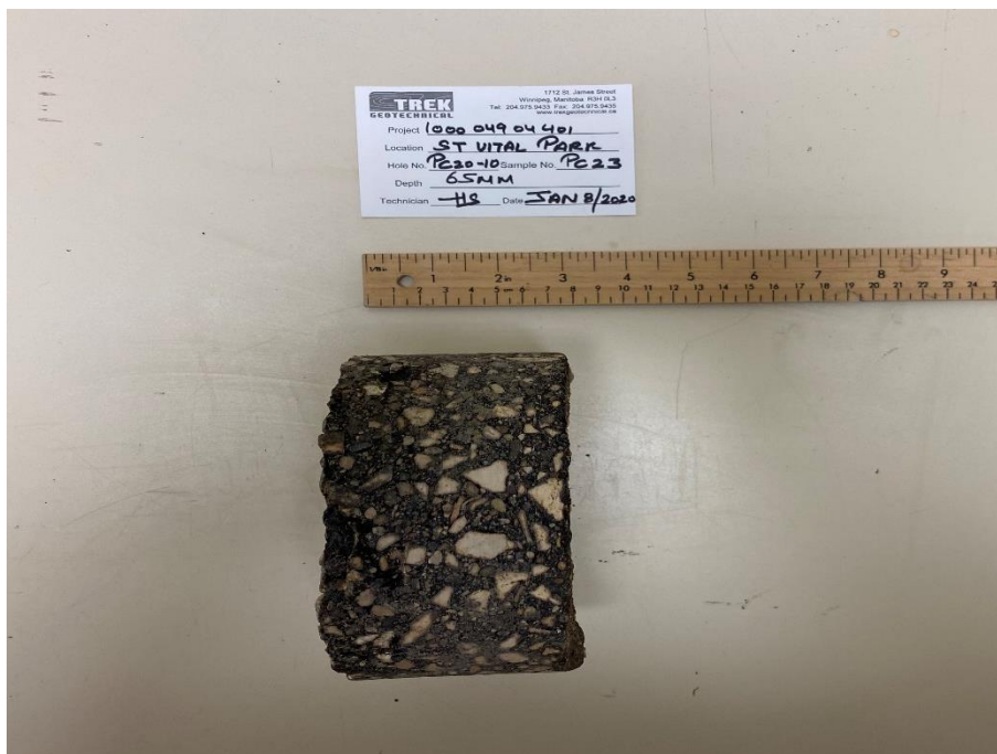
Photo 10: Pavement Core Sample at Pavement Hole PC20-10
