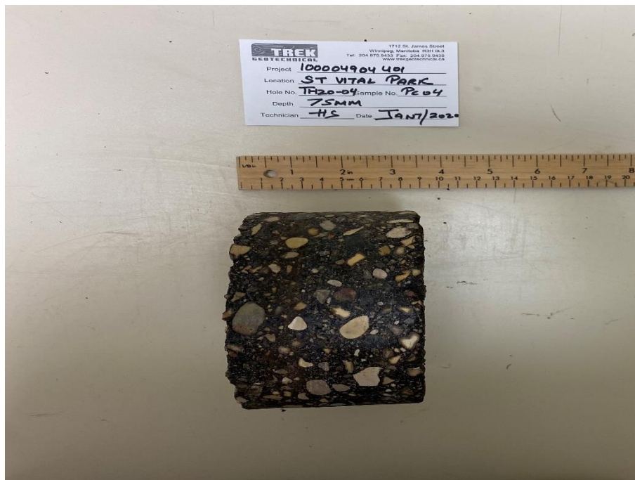
Photo 4: Pavement Core Sample at Test Hole TH20-04
