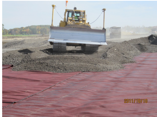
Image 4 – Spreading aggregate over geosynthetic
