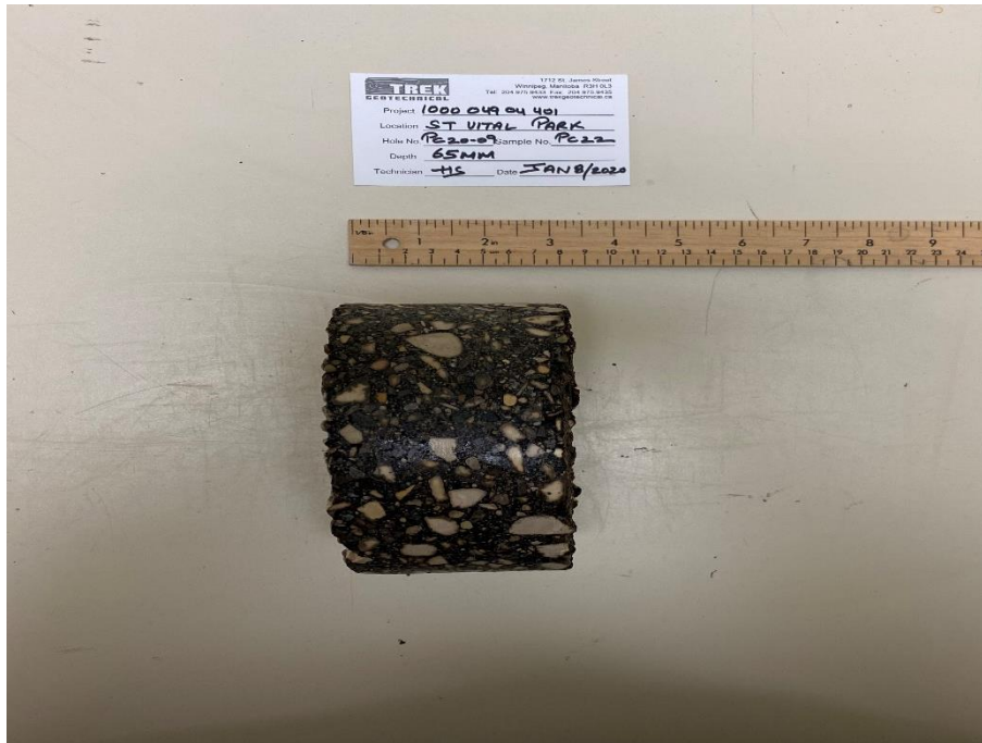
Photo 9: Pavement Core Sample at Pavement Hole PC20-09
