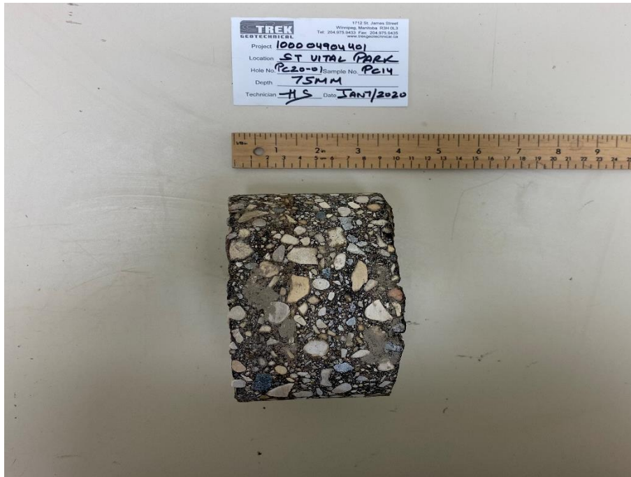
Photo 1: Pavement Core Sample at Pavement Hole PC20-14
