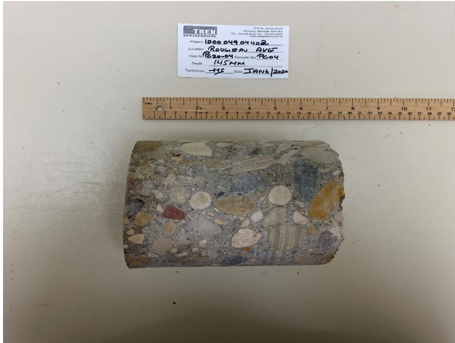
Photo 1: Pavement Core Sample at Pavement Hole PC20-04
