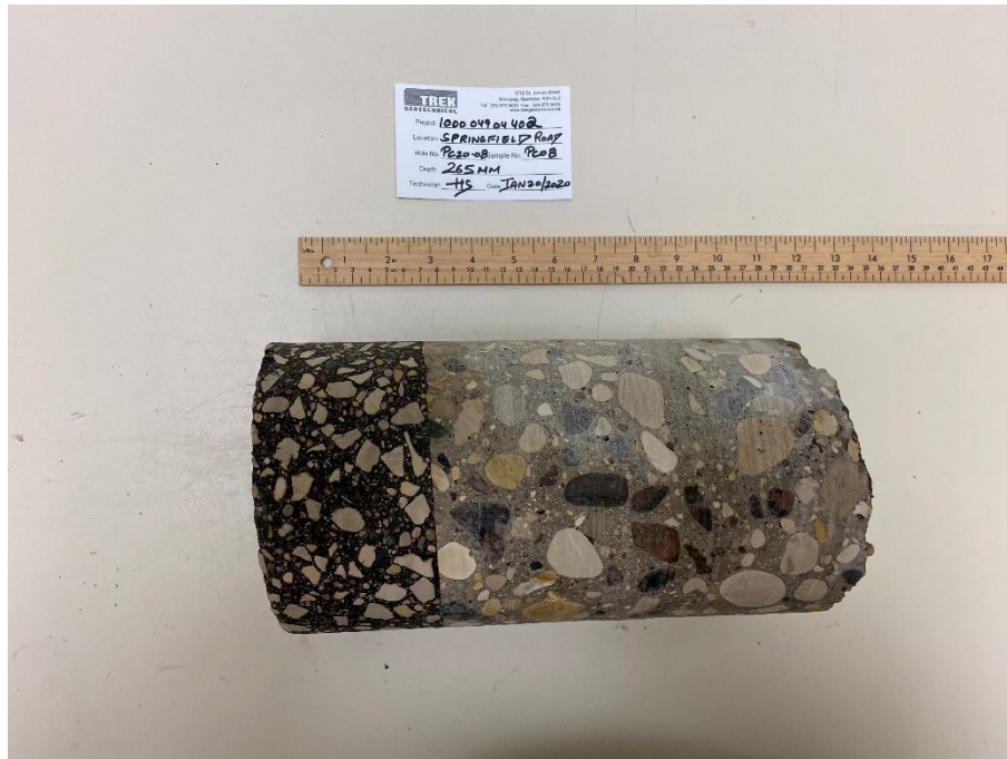
Photo 3: Pavement Core Sample at Pavement Hole PC20-08
