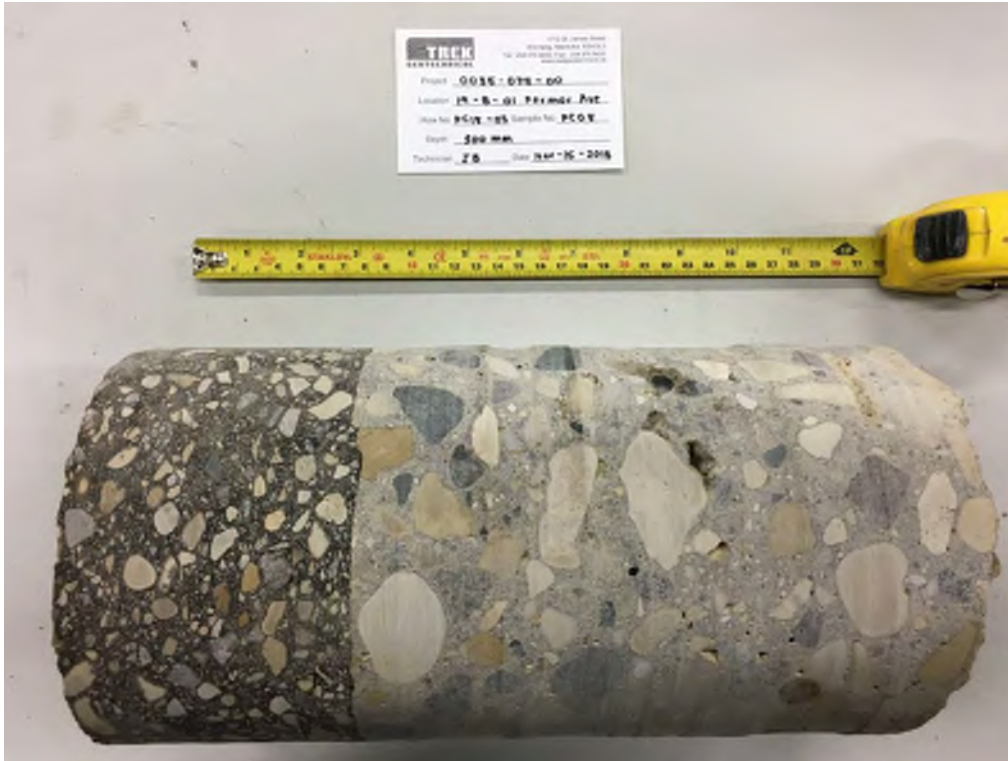
Photo 5: Pavement Core Sample at Test Hole TH18-05
