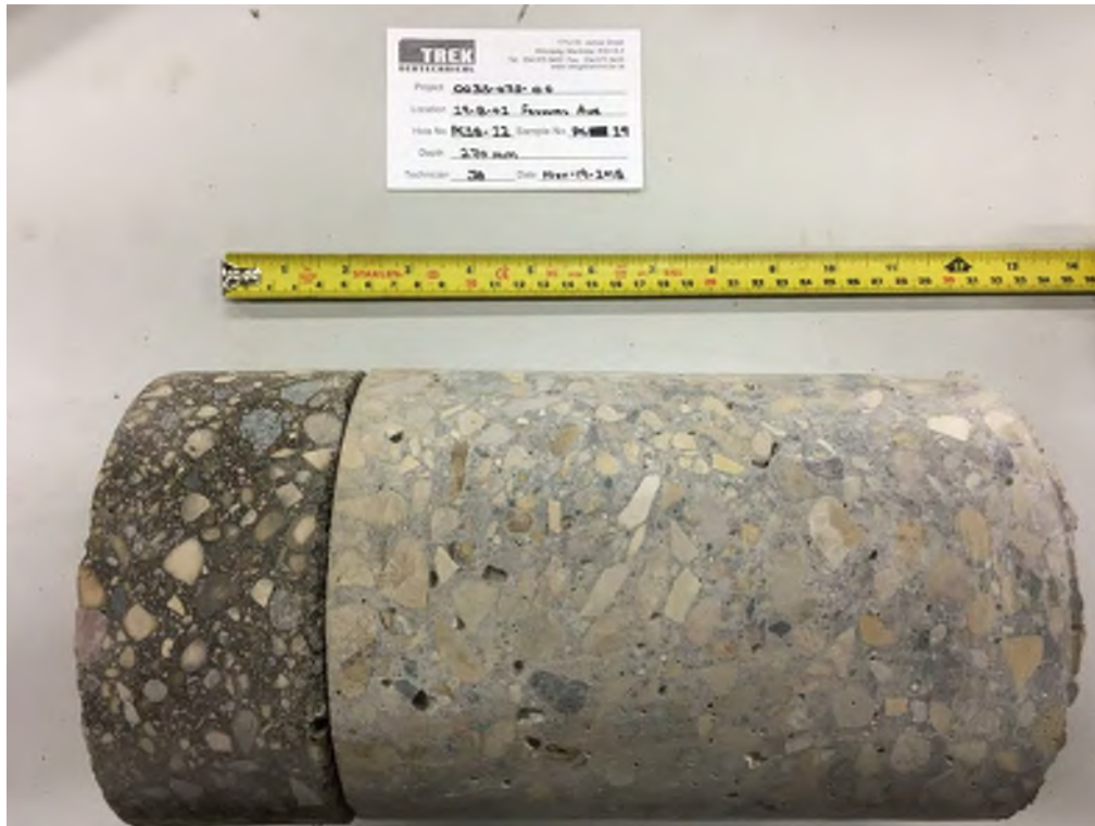
Photo 11: Pavement Core Sample at Test Hole TH18-12
