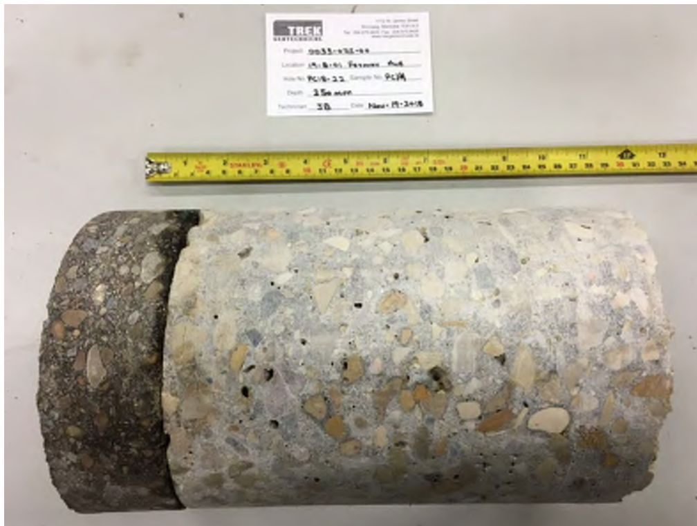
Photo 16: Pavement Core Sample at Test Hole TH18-22
