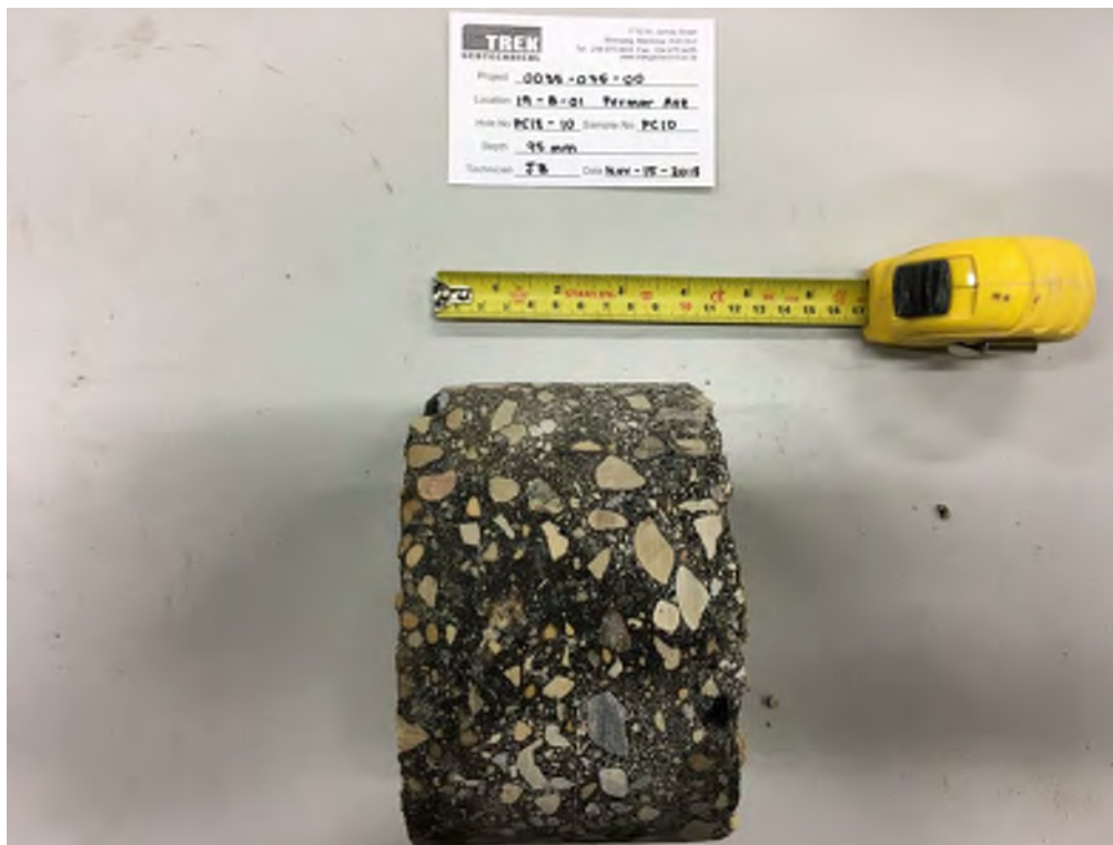
Photo 10: Pavement Core Sample at Test Hole TH18-10
