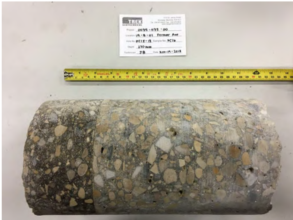
Photo 14: Pavement Core Sample at Test Hole TH18-18
