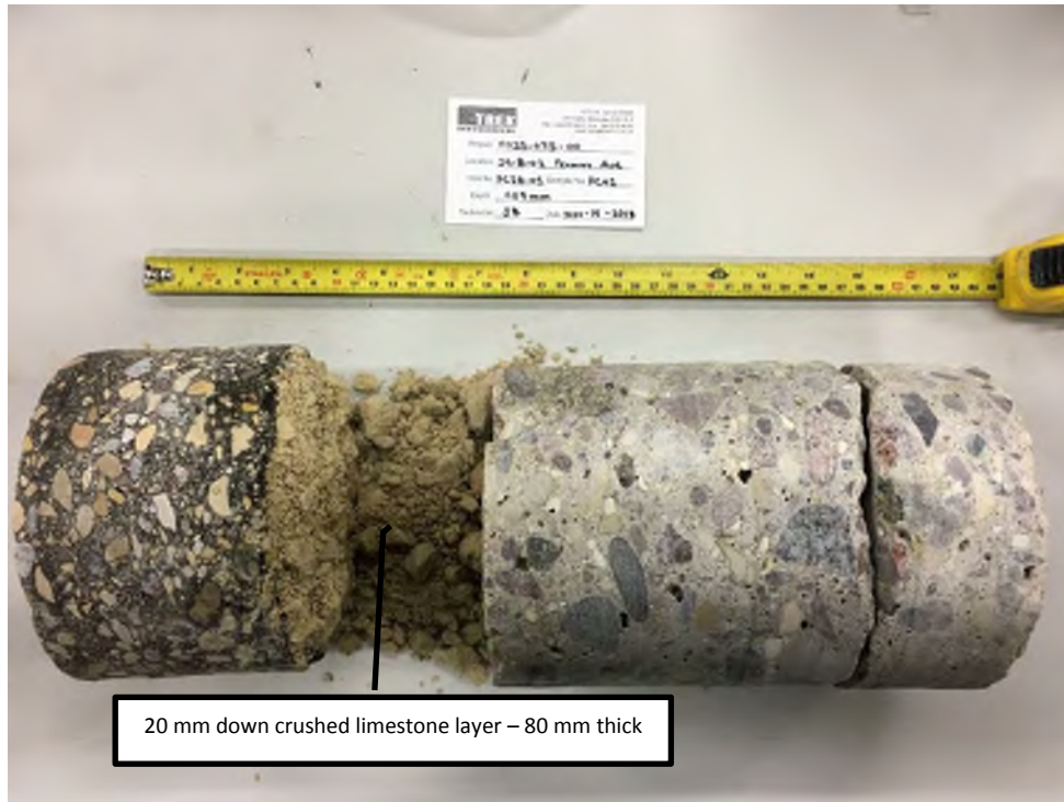
Photo 1: Pavement Core Sample at Test Hole TH18-01
