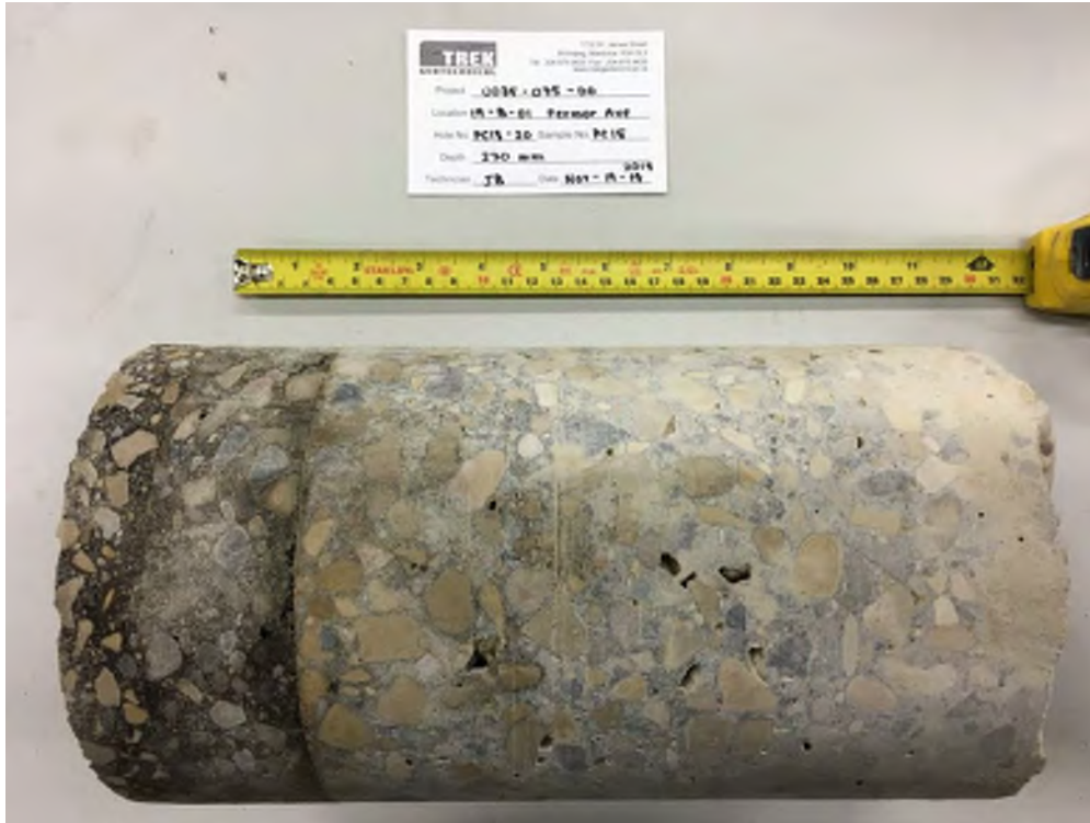
Photo 15: Pavement Core Sample at Test Hole TH18-20
