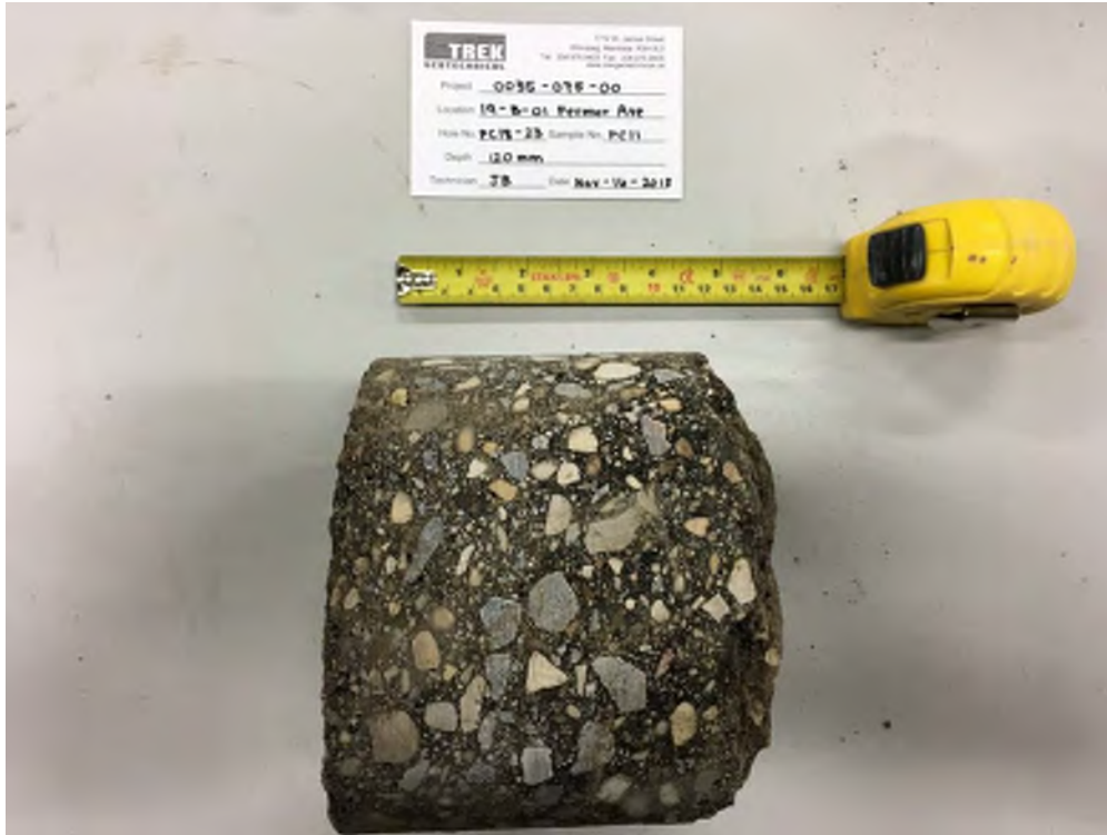
Photo 17: Pavement Core Sample at Test Hole TH18-23
