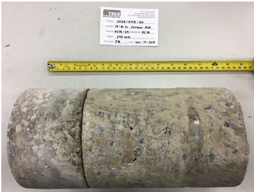
Photo 18: Pavement Core Sample at Test Hole TH18-24
