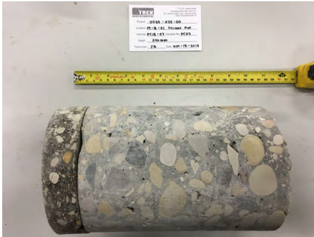
Photo 7: Pavement Core Sample at Test Hole TH18-07
