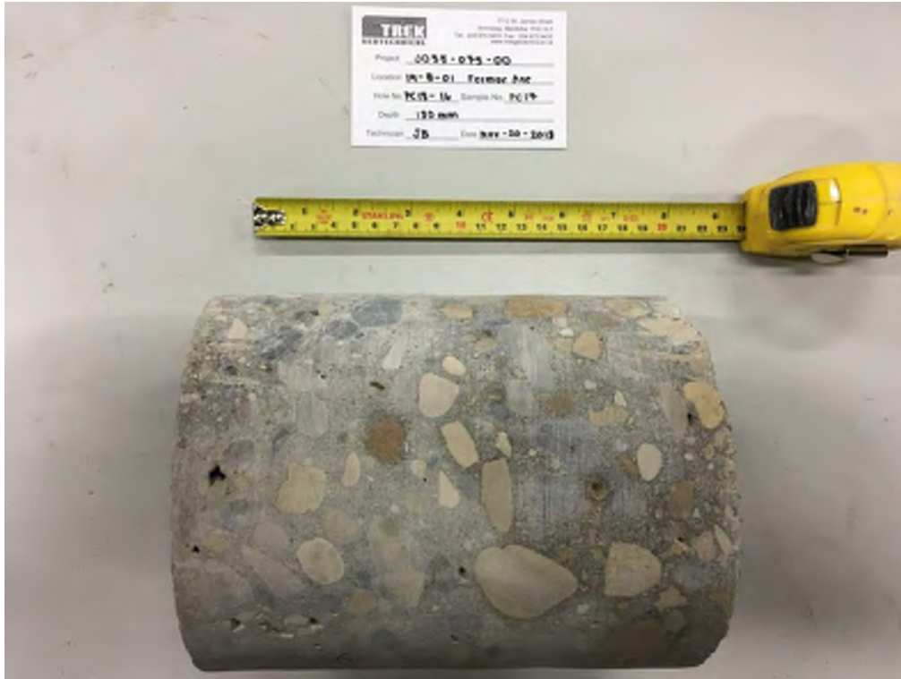
Photo 13: Pavement Core Sample at Test Hole TH18-16
