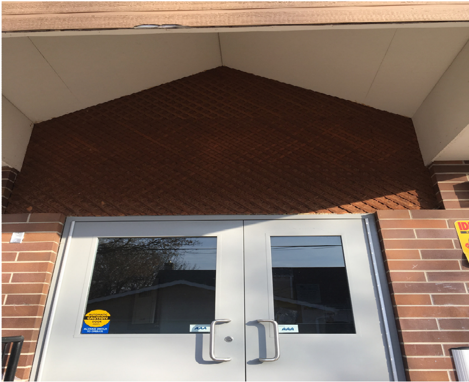
Figure 7: New siding & vented soffit throughout.
