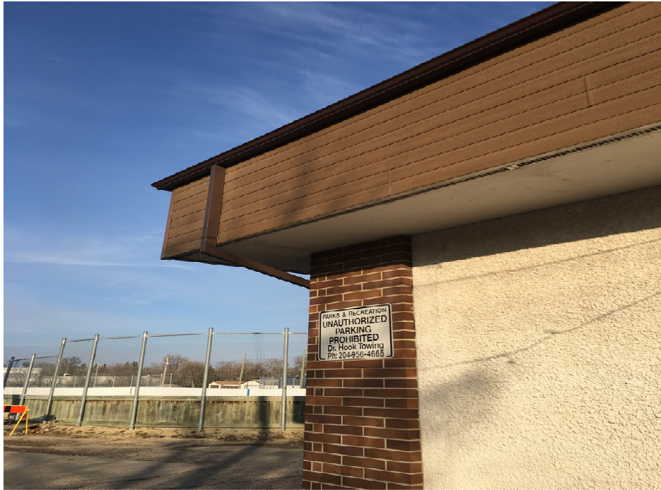
Figure 6: Match existing CanExcel Siding.
