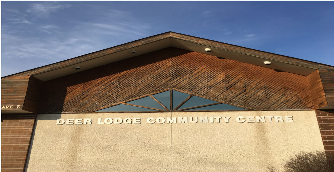
Figure 8: New siding & vented soffit throughout.
