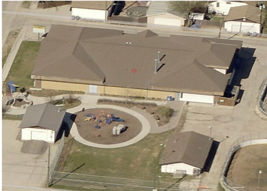
Figure 1: VIEW FROM EAST ELEVATION
