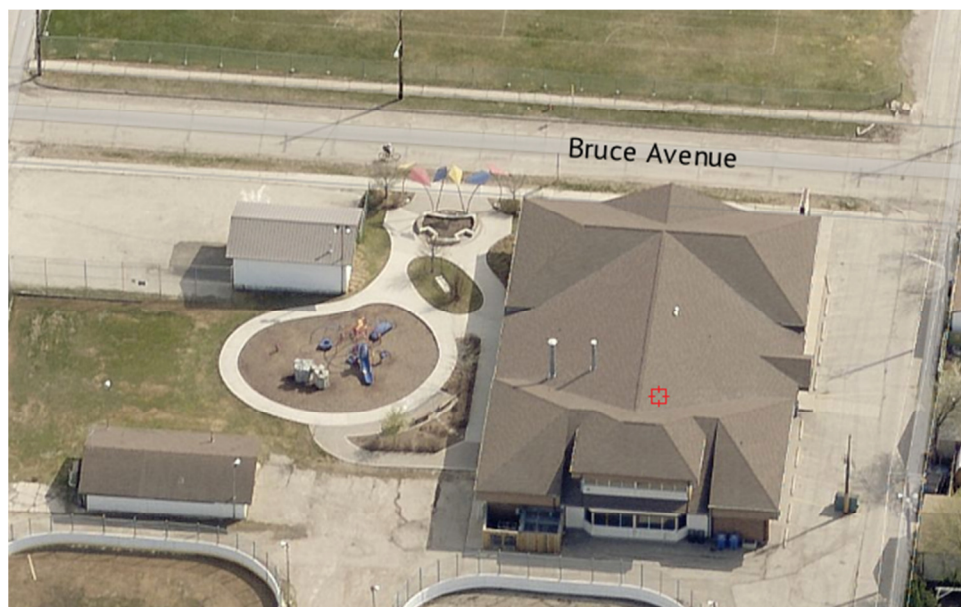
Figure 2: VIEW FROM NORTH ELEVATION
