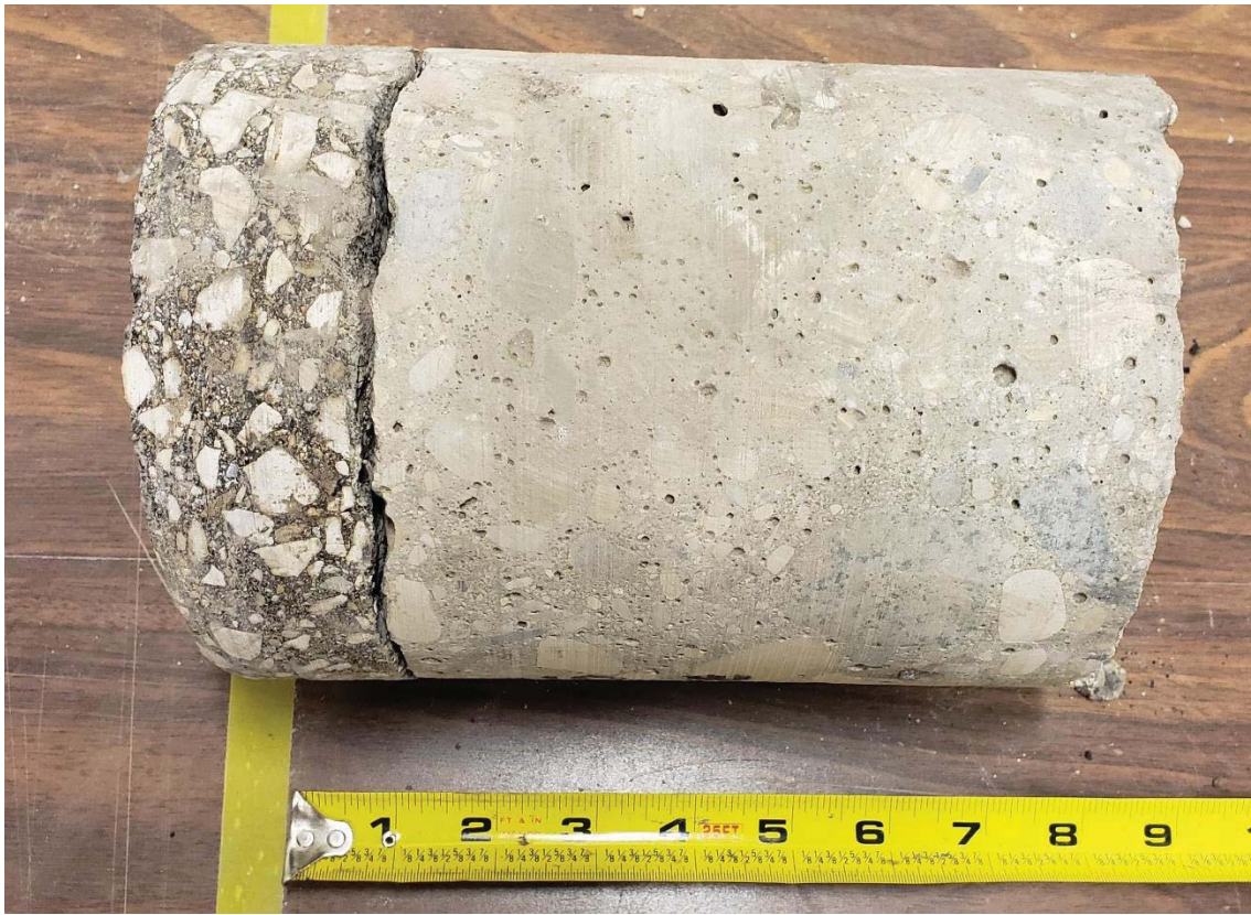
Figure 5 – PC-11 Lodge Ave
