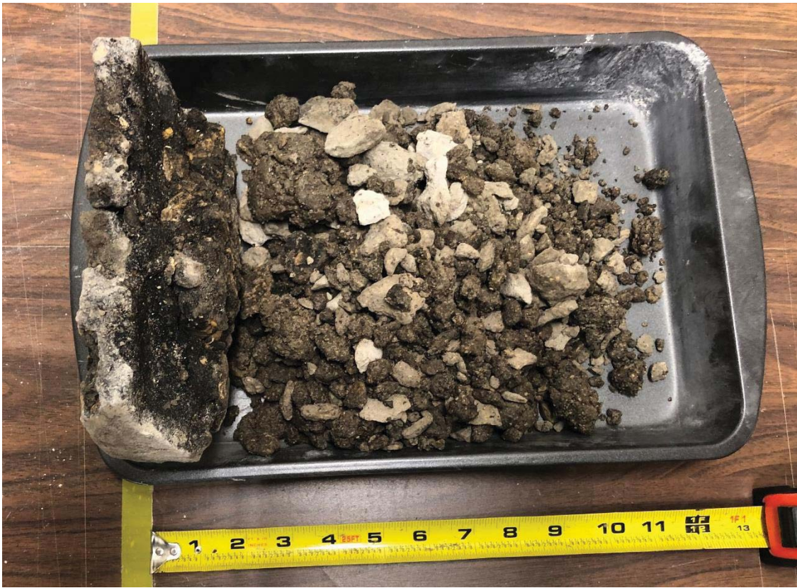
Figure 1 – TH-05 Strathcona Ave (asphalt and broken concrete, actual core depth 120 mm)
