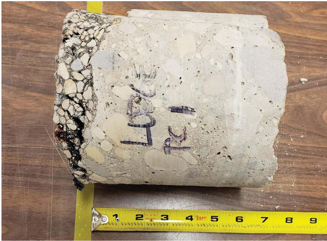
Figure 1 – PC-07 Lodge Ave
