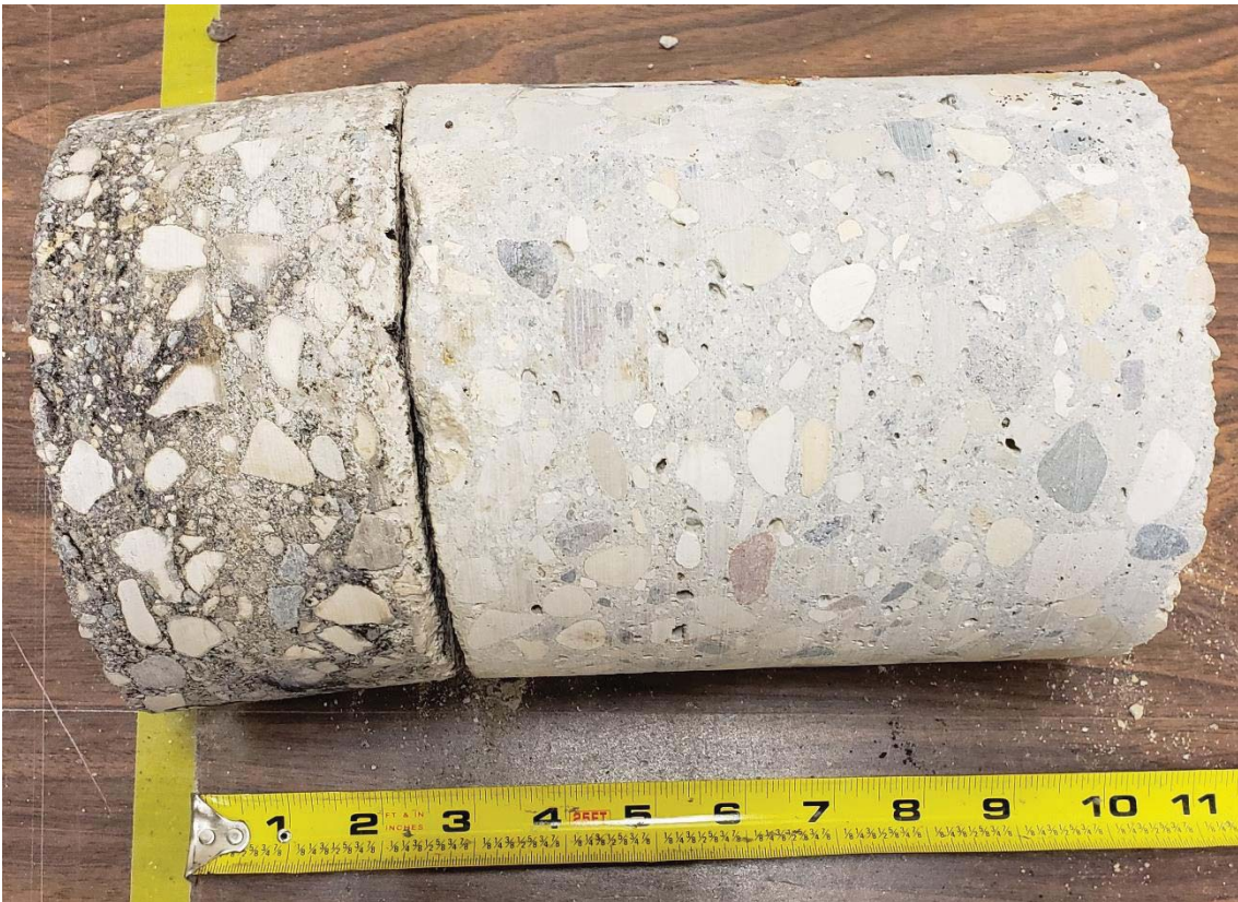
Figure 8 – PC-14 Lodge Ave
