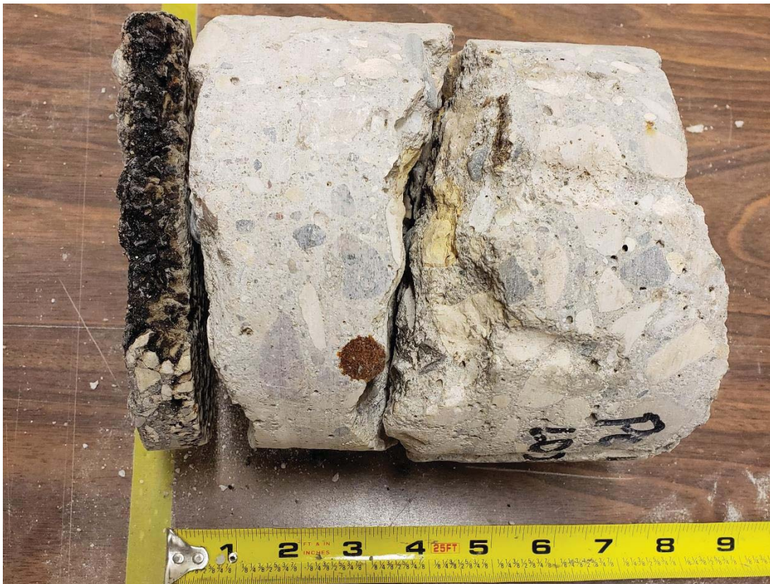
Figure 4 – PC-10 Lodge Ave
