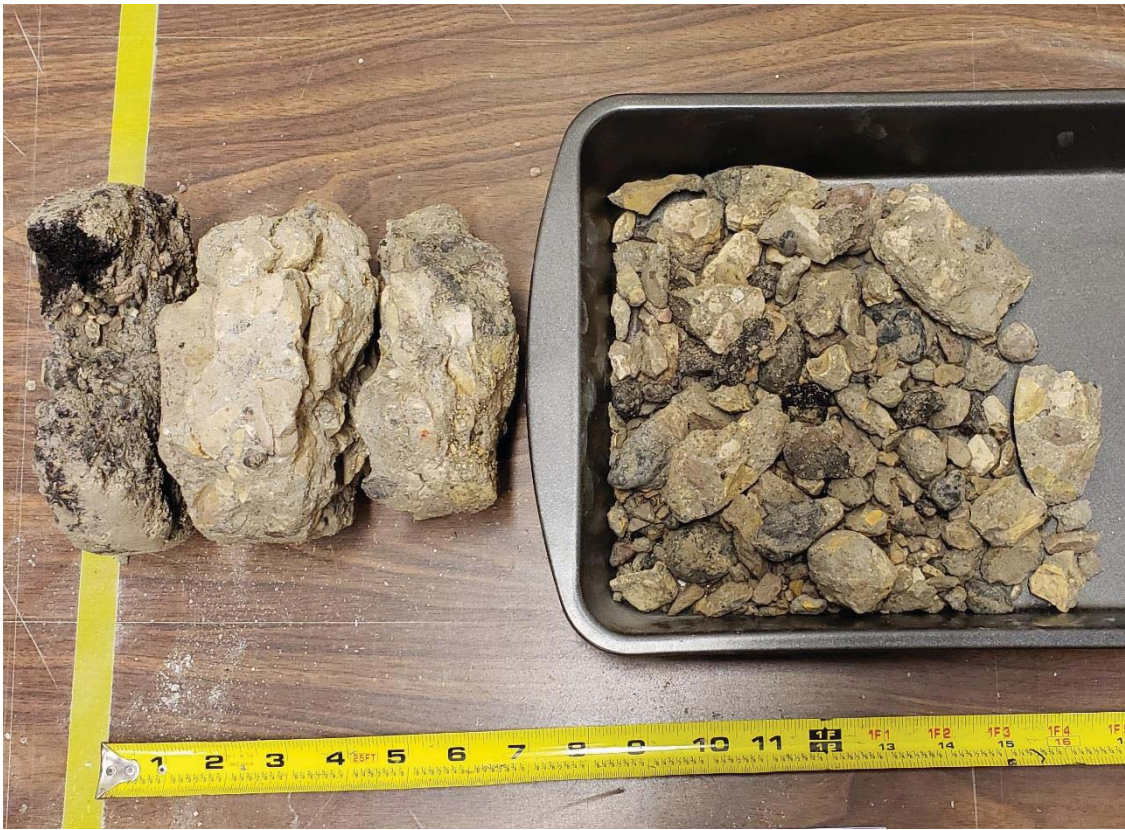
Figure 1 – PC-01 Ainslie St (asphalt and broken concrete, actual core depth 240 mm)
