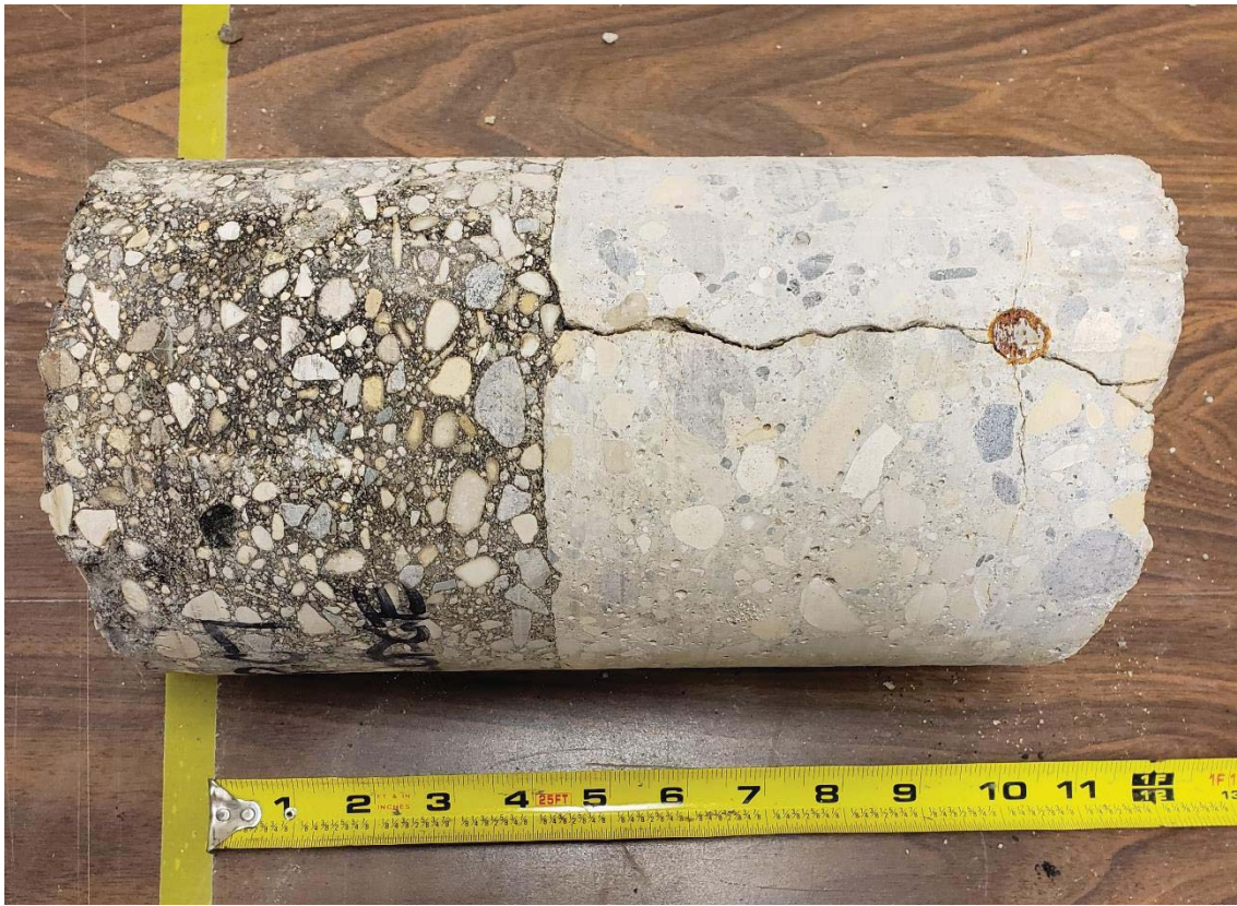
Figure 7 – PC-13 Lodge Ave
