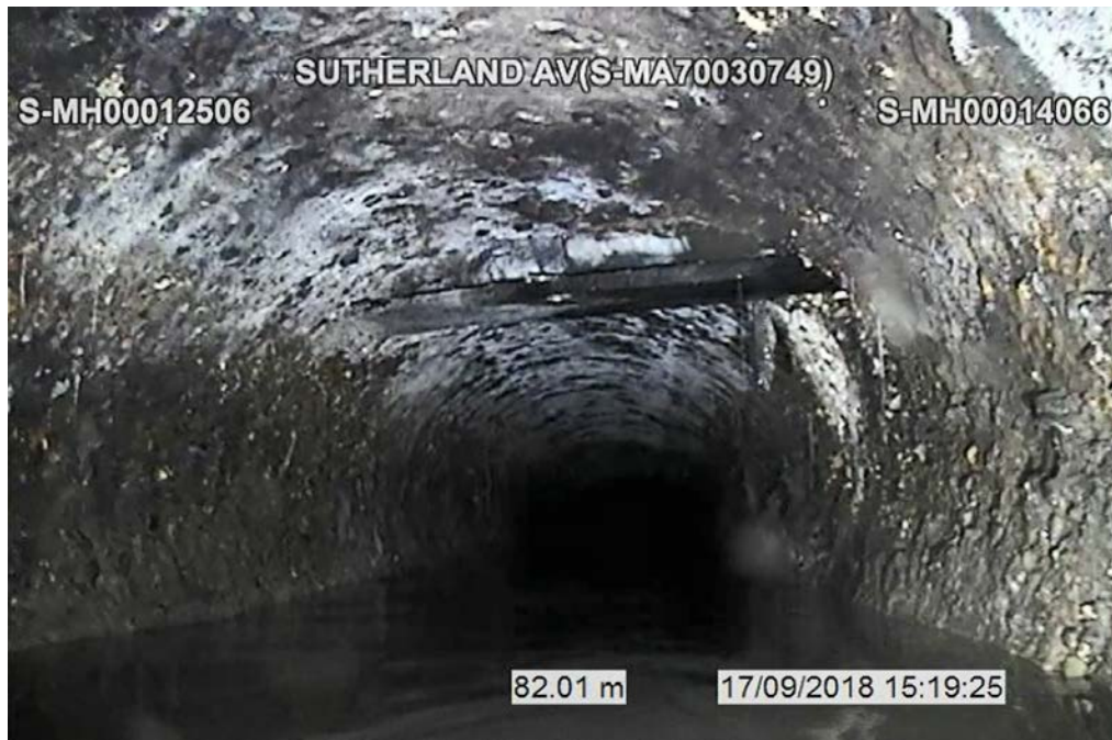
Figure 18 – Sheet 24, Dwg 12288, S-MA70030750 (Sutherland Av.) – 150 mm Watermain Crossbore at 94 m Downstream.
