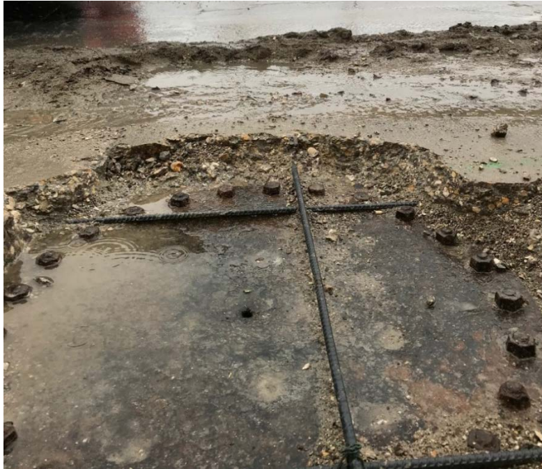
Figure 3: Sheet 3, Dwg 12267, Flanged Access Point in sidewalk on S-MA70012139 on McPhillips St.
