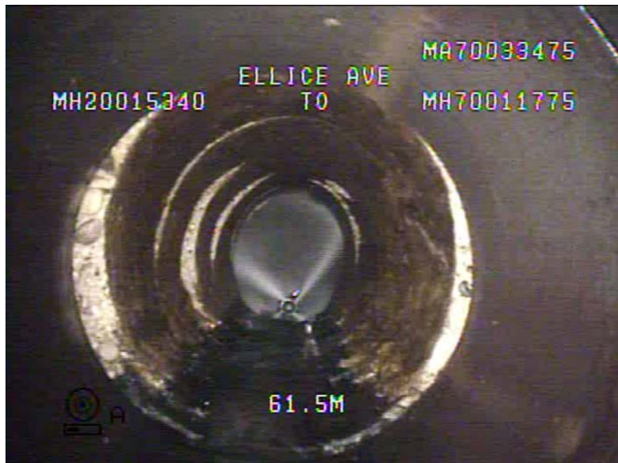
Figure 8 – Sheet 6, Dwg 12270, S-MA70033475 (Ellice Av.) – Material and Cross Section Change to Oval Precast Concrete.
