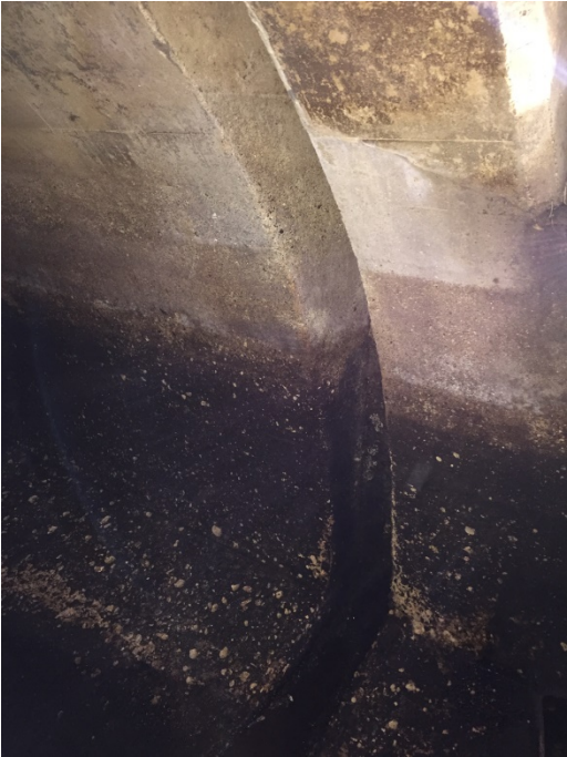
Photograph 15. ↑ Mile 64.14 – Existing Groove (Side of Aqueduct)
