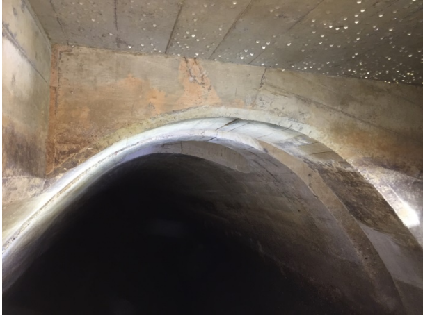
Photograph 14. ↑ Mile 64.14 – Existing Groove (Top of Aqueduct)
