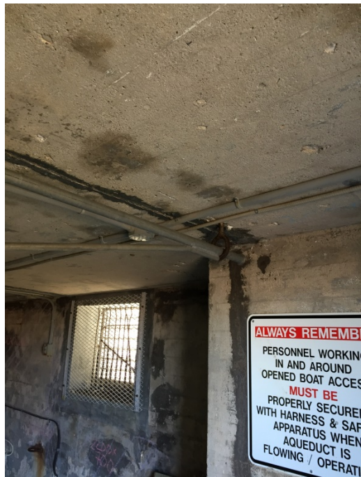
Photograph 4. ↑ Mile 17.05 – Boathouse Interior Wall and Roof
