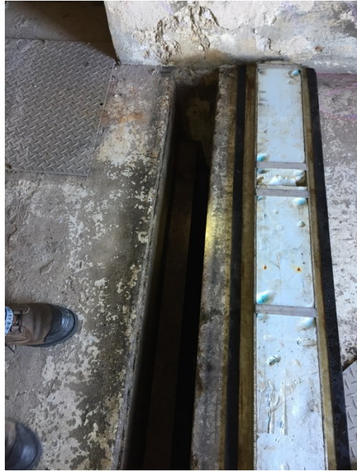
Photograph 2. ↑ Mile 17.05 – Existing Stop Log Opening and Cover
