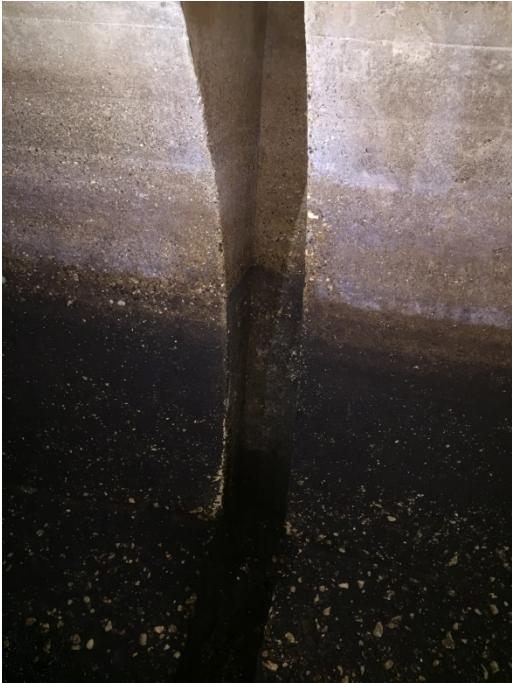
Photograph 16. ↑ Mile 64.14 – Existing Groove (Side of Aqueduct)
