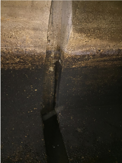
Photograph 21. ↑ Mile 73.69 – Existing Groove (Side of Aqueduct)
