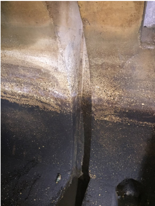
Photograph 24. ↑ Mile 73.69 – Existing Groove (Side of Aqueduct)
