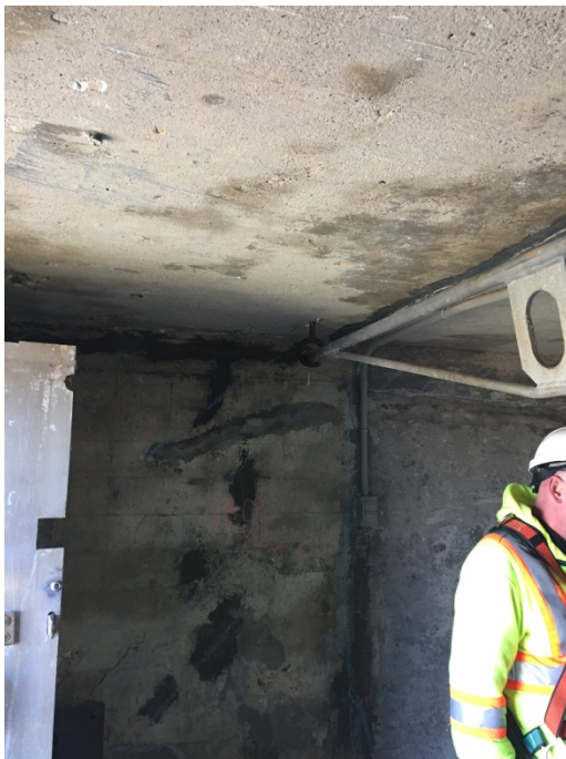
Photograph 3. ↑ Mile 17.05 – Boathouse Interior Wall and Roof
