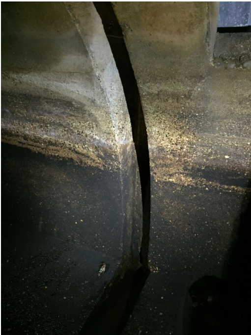
Photograph 23. ↑ Mile 73.69 – Existing Groove (Side of Aqueduct)
