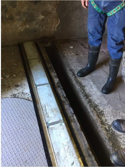
Photograph 1. ↑ Mile 17.05 – Existing Stop Log Opening and Cover
