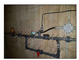
REMOVE EXISTING SEAL WATER PIPING, VALVES AND ACCESSORIES AS PER SEAL WATER DEMOLITION SCHEMATIC DIAGRAM ON DRAWING M-02
