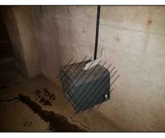
REMOVE EXISTING UNIT HEATER C/W SUPPORTING BRACKETS
