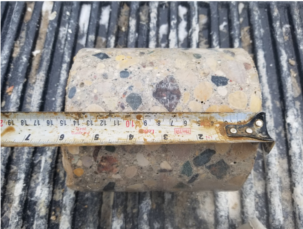
Photograph 24: Test Hole CH19-44 - Thatcher Drive
