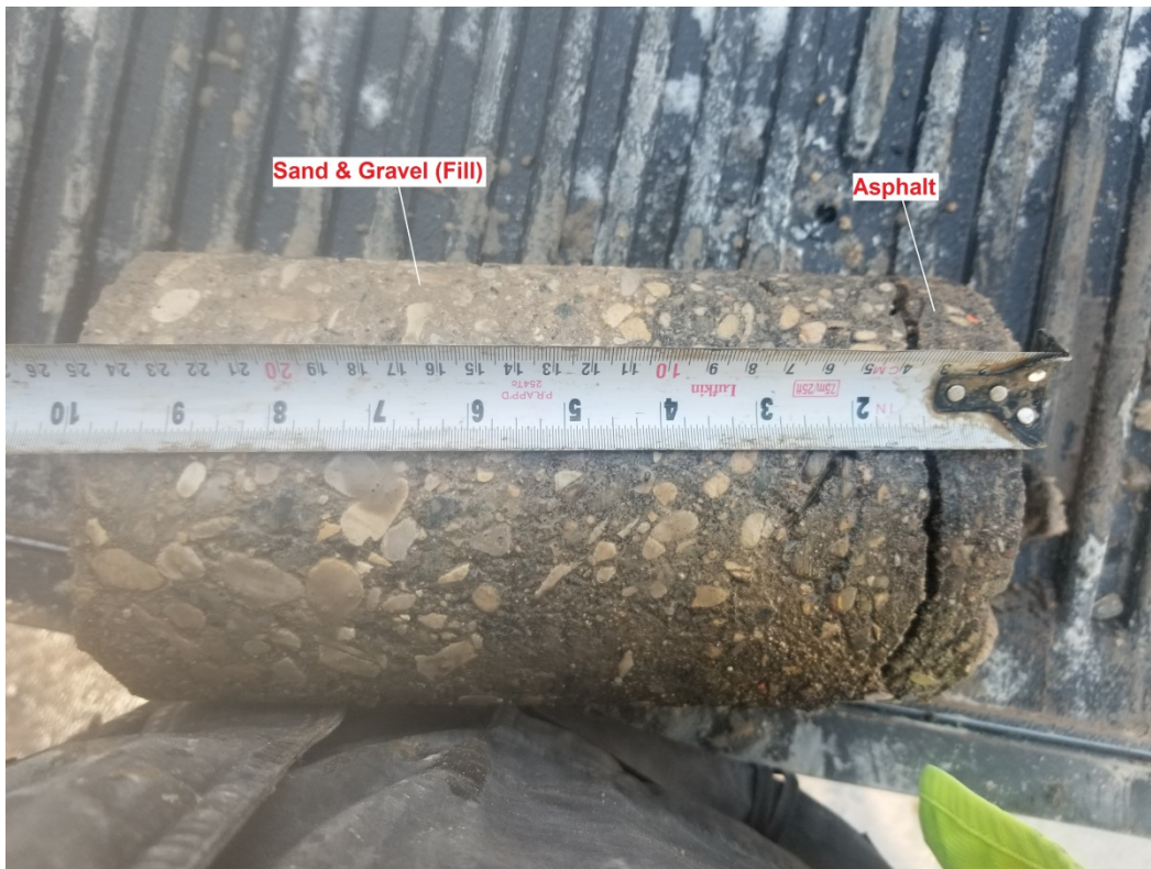
Photograph 10: Test Hole TH19-12 - Hudson Street
