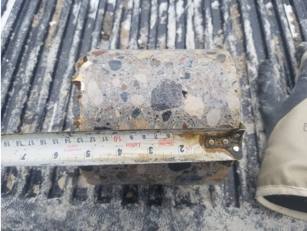
Photograph 17: Test Hole CH19-37 - Caledon Road
