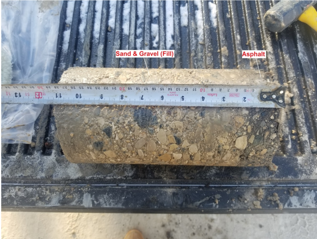
Photograph 9: Test Hole TH19-11 - Hudson Street
