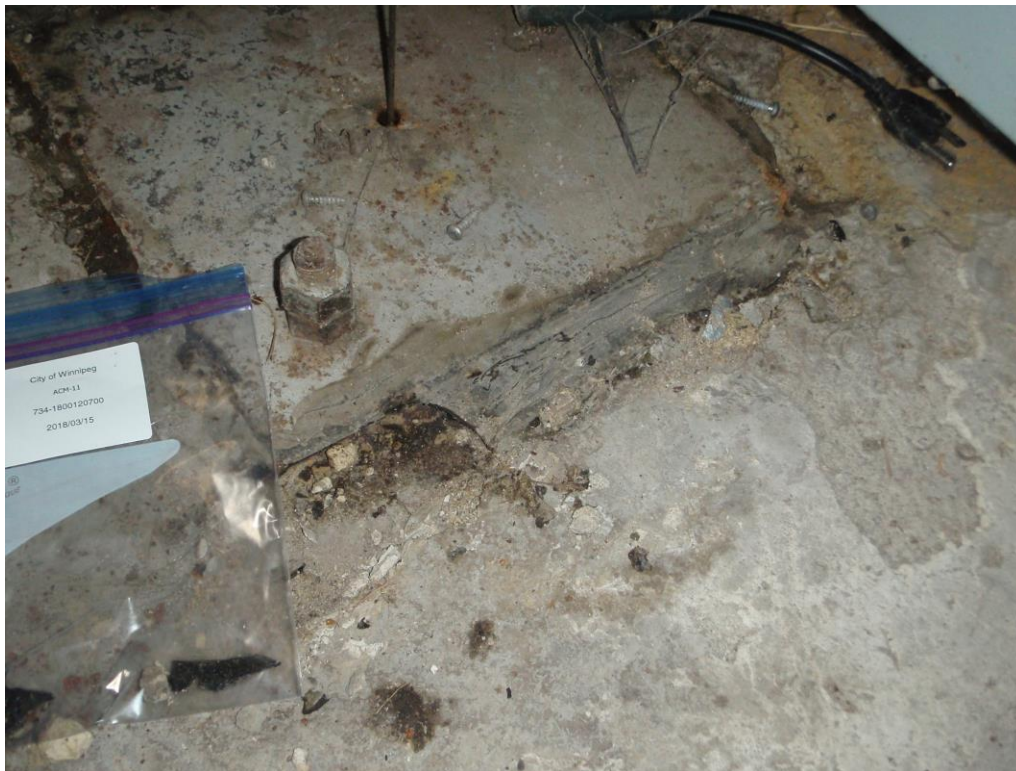
Photo 46: General view of condition of the sealant found to contain asbestos around the metal plate for the wet well float level on the floor of the main level along the north wall. (March 15, 2018)
