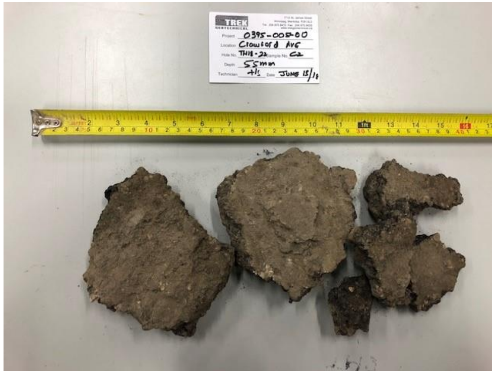
Photo 1: Pavement Core Sample at Test Hole TH18-22
