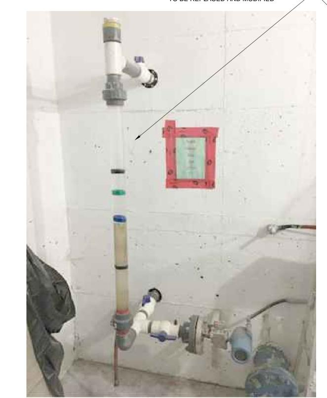
EXISTING DP LEVEL MEASUREMENT SYSTEM TO BE REPLACED AND MODIFIED
