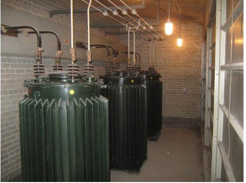
Photograph:3-5Description:2400V/600V, 333kVA single phase transformers within the vault.Date:May 4, 2010
