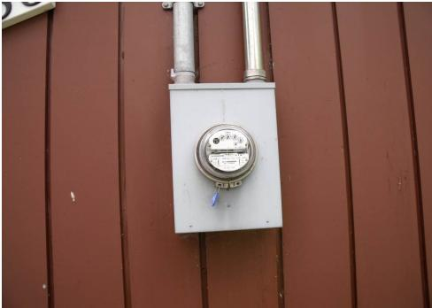
Photograph:3-2Description:120/240V Hydro service meter mounted on the north side of the station.Date:June 2, 2009
