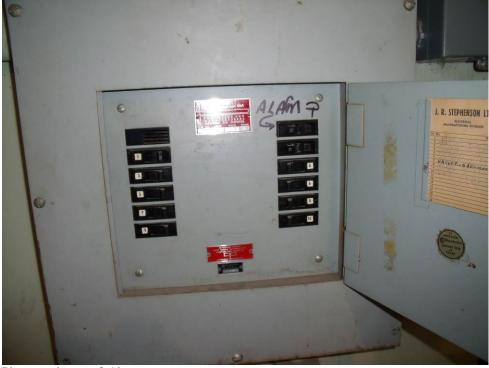
Photograph:3-19Description:120/240V 12 circuit distribution panelDate:June 2, 2009
