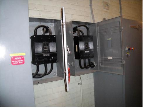
Photograph:3-14Description:Two flood pump ITE feeder breakers mounted beside their corresponding RVS cabinetsDate:June 2, 2009
