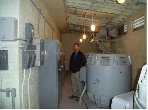
Photograph:3-9Description:View showing limited space between the soft starter and the pumps.Date:June 2, 2009
