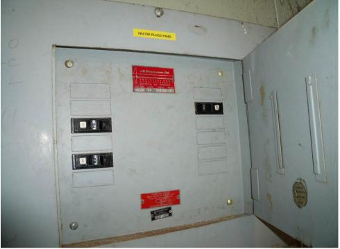
Photograph: Description: Date: 3-21 120/240V heater distribution panel June 2, 2009
