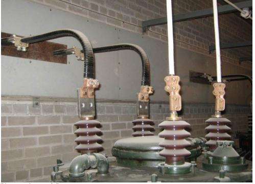
Photograph:3-7Description:2400V/600V, 333kVA single phase transformers connected to the 600V delta bus.Date:May 4, 2010
