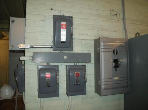
Photograph:3-10Description:60A 600V distribution and one ITE flood pump feeder breaker.Date:June 2, 2009
