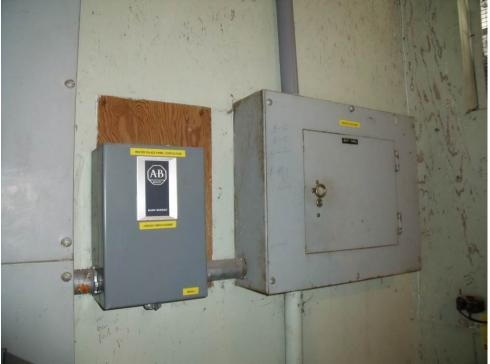
Photograph:3-20Description:120/240V heater distribution panel and thermostat control contact cabinetDate:June 2, 2009
