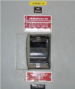
Photograph:3-18Description:Main 200A breaker for the 120/240V distribution equipmentDate:June 2, 2009
