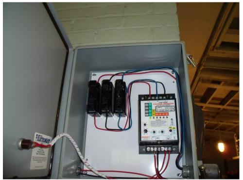
Photograph:3-22Description:600V power monitoring equipmentDate:June 2, 2009
