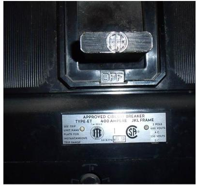
Photograph:3-13Description:Flood pump ITE feeder breaker name plateDate:June 2, 2009
