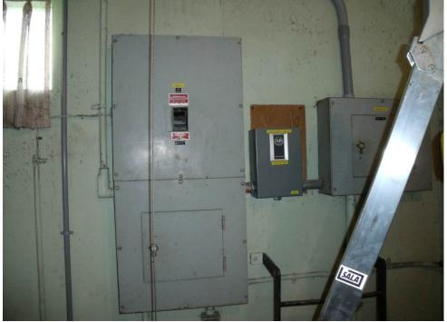
Photograph:3-17Description:120/240V distribution equipment on mounted north wall of the stationDate:June 2, 2009
