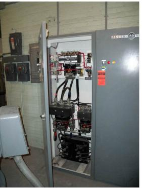
Photograph:3-11Description:View showing that the RVS door cannot open to its full range.Date:June 2, 2009
