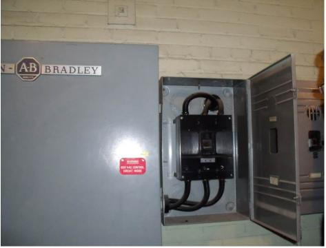
Photograph:3-12Description:Flood pump ITE feeder breaker mounted beside its corresponding RVSDate:June 2, 2009
