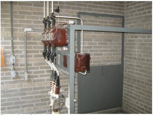
Photograph:3-6Description:Hydro service metering CT's and PT's within the vault.Date:May 4, 2010
