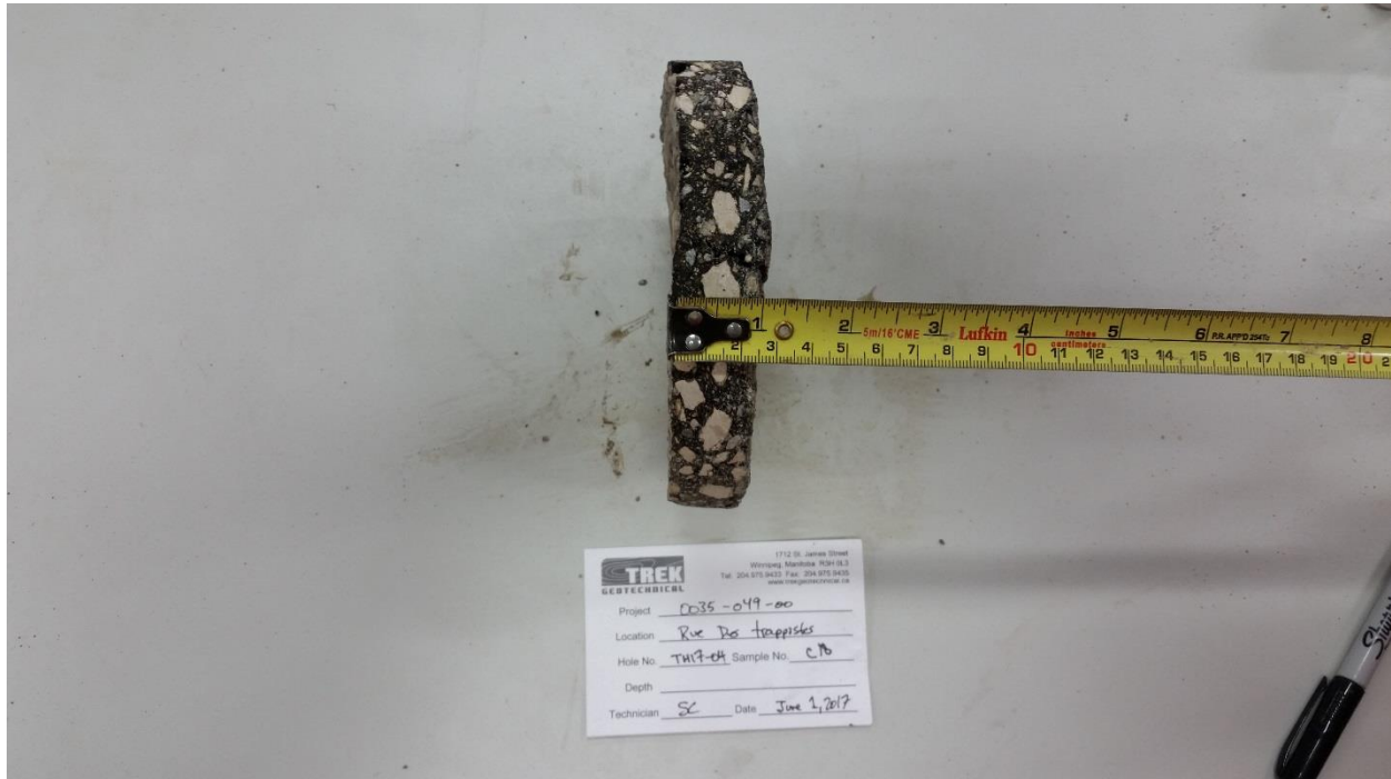
Photo 4: Pavement Core Sample at Test Hole TH17-04
