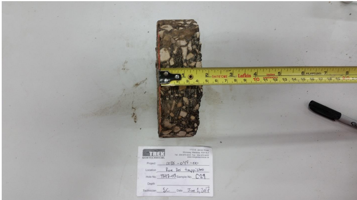
Photo 3: Pavement Core Sample at Test Hole TH17-03
