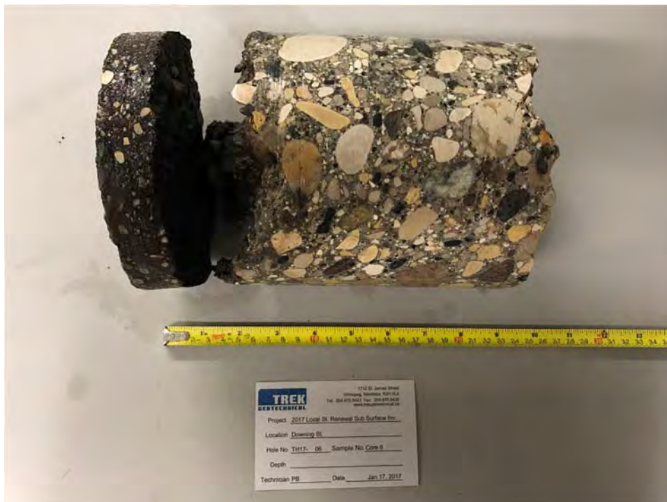
PHOTO 6: DOWNING STREET PAVEMENT CORE AT TEST HOLE TH17-06
