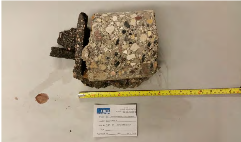
PHOTO 1: DOWNING STREET SPAVEMENT CORE AT TEST HOLE TH17-01
