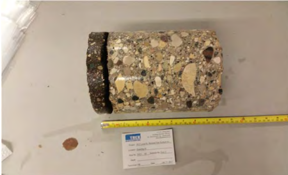
PHOTO 3: DOWNING STREET PAVEMENT CORE AT TEST HOLE TH17-03
