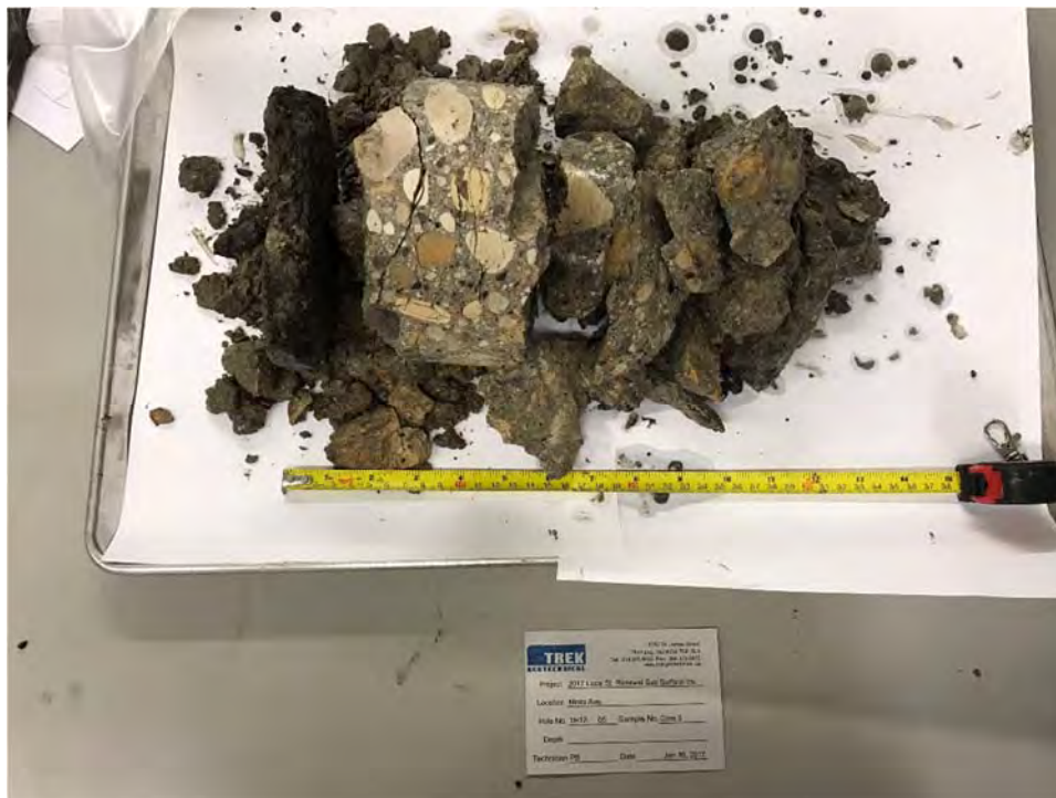
PHOTO 5: MINTO STREET PAVEMENT CORE AT TEST HOLE TH17-05
