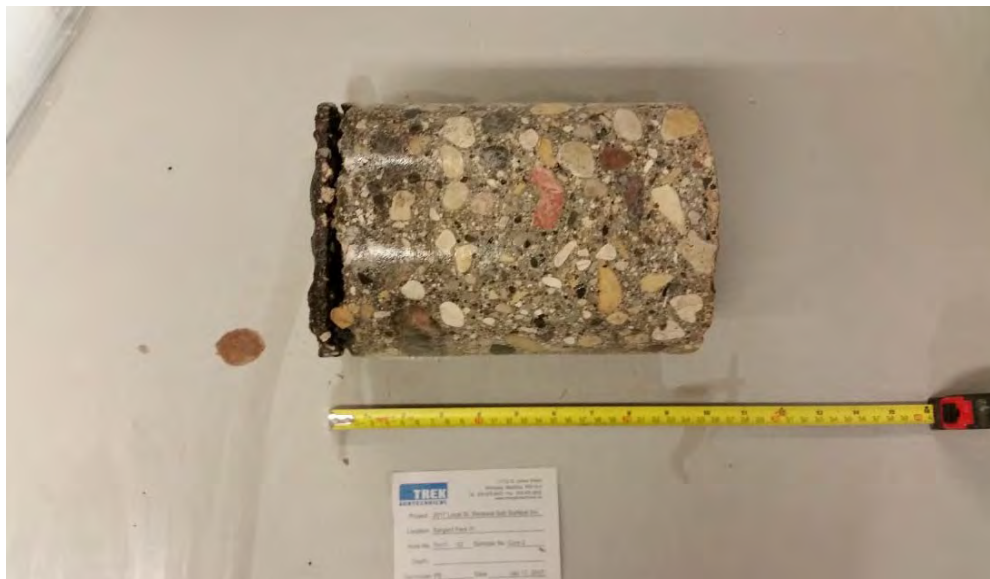
PHOTO 2: DOWNING STREET PAVEMENT CORE AT TEST HOLE TH17-02
