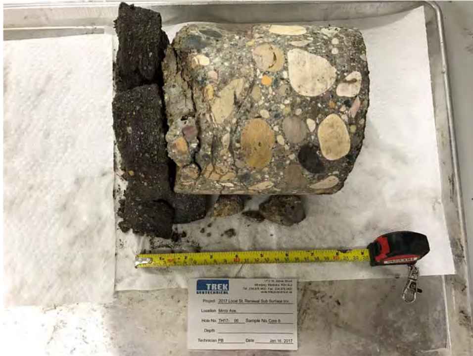
PHOTO 6: MINTO STREET PAVEMENT CORE AT TEST HOLE TH17-06
