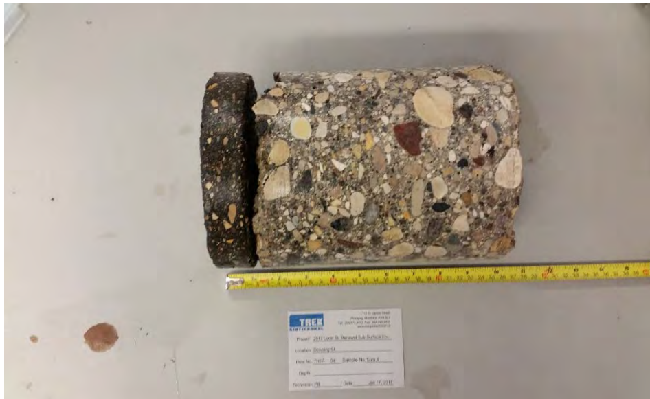
PHOTO 4: DOWNING STREET PAVEMENT CORE AT TEST HOLE TH17-04
