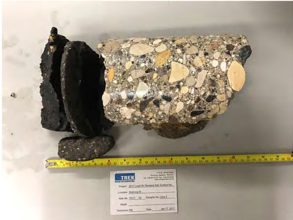
PHOTO 5: DOWNING STREET PAVEMENT CORE AT TEST HOLE TH17-05
