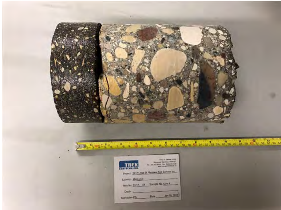
PHOTO 4: MINTO STREET PAVEMENT CORE AT TEST HOLE TH17-04
