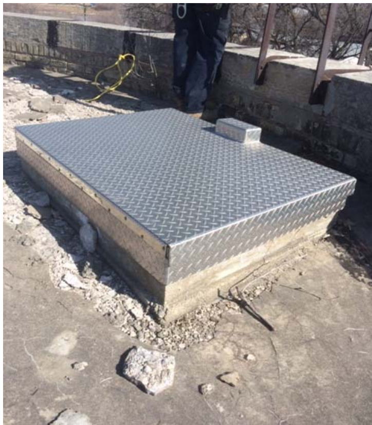
Add: Photo 10: Surge Tower Roof Hatch
