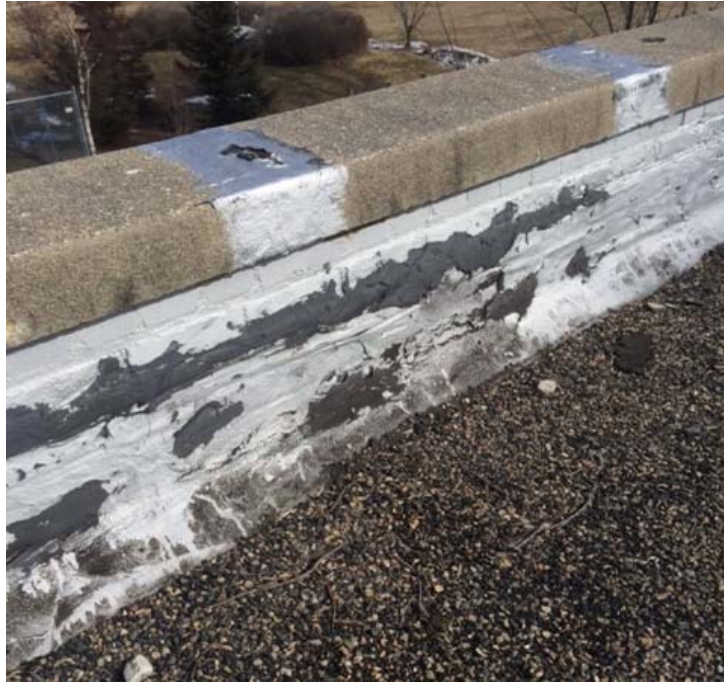
Add: Photo 1: Tache Booster Pumping Station Roof
