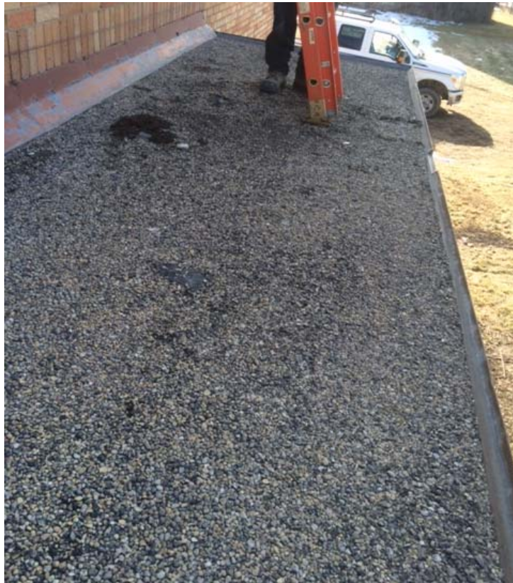
Add: Photo 2: Tache Booster Pumping Station Roof
