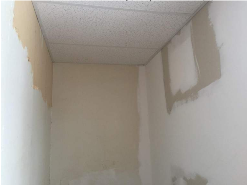
Photo 6. Second floor hallway, acoustic tiles.
