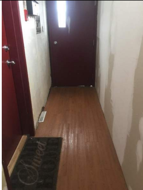
Photo 3. First Floor Hallway
