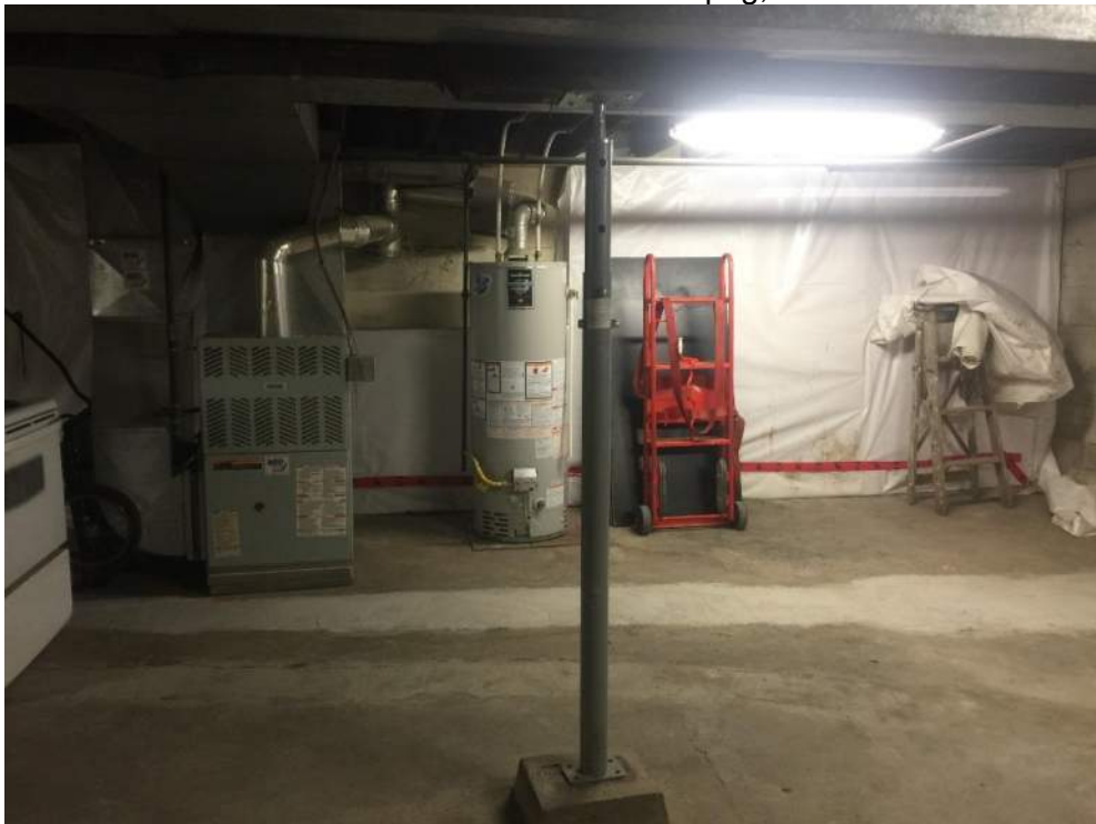
Photo 2. Unfinished Basement with utilities.
