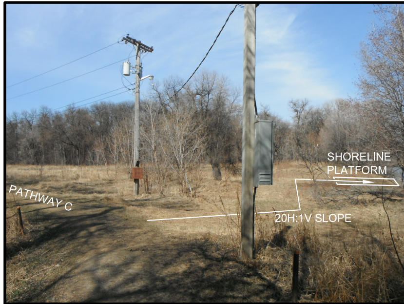
PHOTOGRAPH 1: FACING NORTHWEST SHOWING APPROXIMATE LOCATION OF PATH AND SHORELINE PLATFORM.
