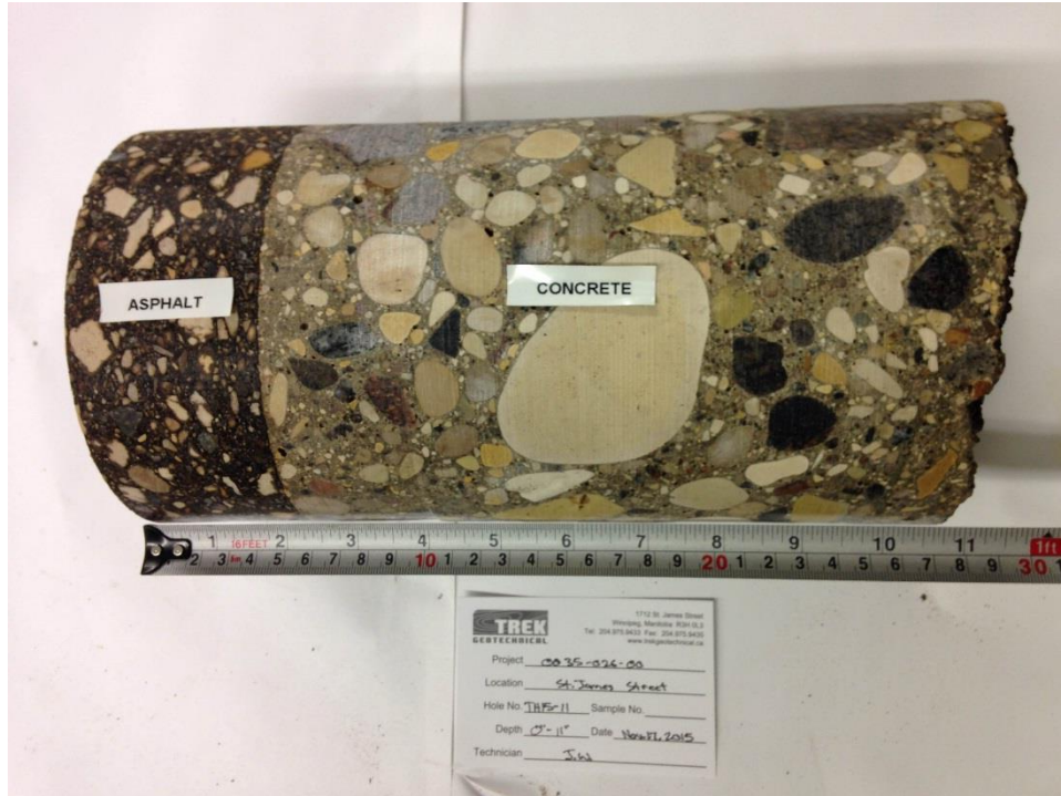
Photo 11: Concrete Core Sample From Test Hole TH15-11
