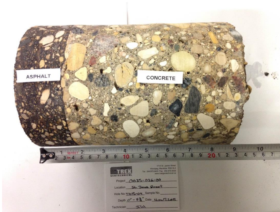
Photo 4: Concrete Core Sample From Test Hole TH15-04
