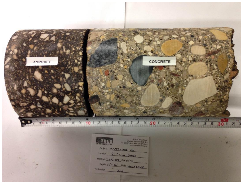
Photo 8: Concrete Core Sample From Test Hole TH15-08
